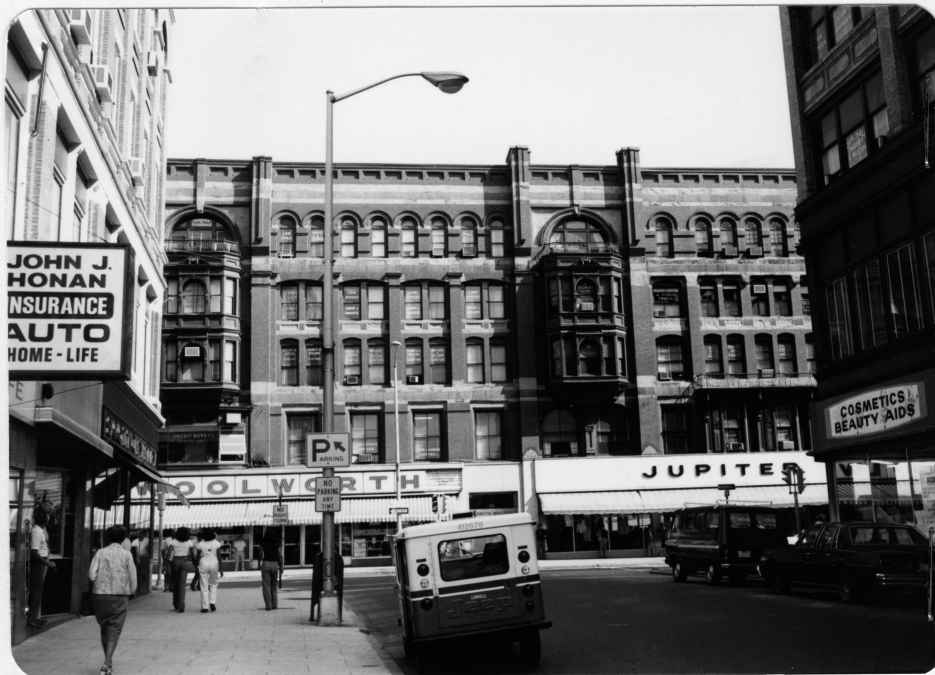
View from: South. Photo taken: June, 1979.
