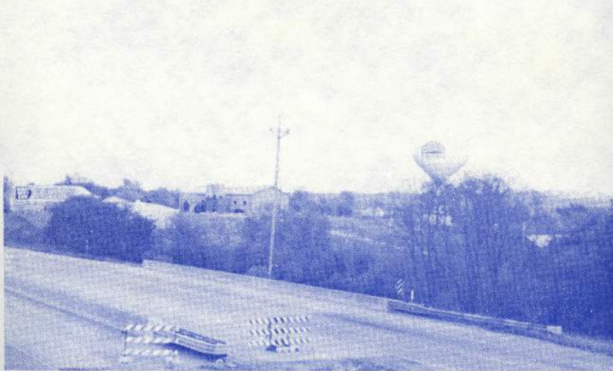
View of the Coralville Water Plant area and Interstate 80 (under construction) from 12th Avenue.
