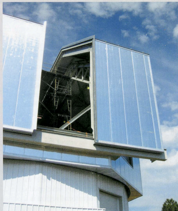
The DCT shutters in the open position, showing the viewing slit.
