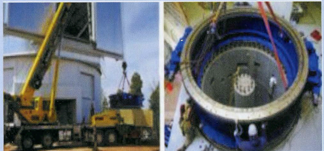
The first of the telescope pieces to go in was the pedestal, shown above being lifted out of its crate (left) and being placed on the bolt pattern (right). Most of the large pieces are being hoisted by crane through the open shutter doors of the dome, and are then lowered into place.
