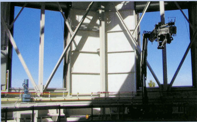
The well-ventilated DCT dome, with personnel lift (at right, sporting copious hydraulics) and motor (blue with white drive wheel housing, lower left).
