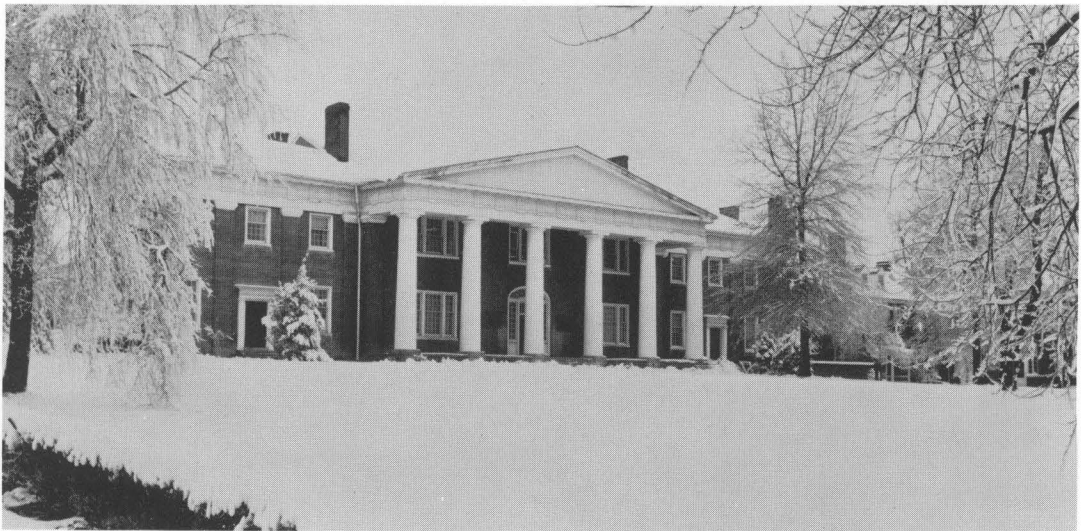
Olde Centre, Administration building
