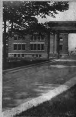
WEST HALL DRIVE
