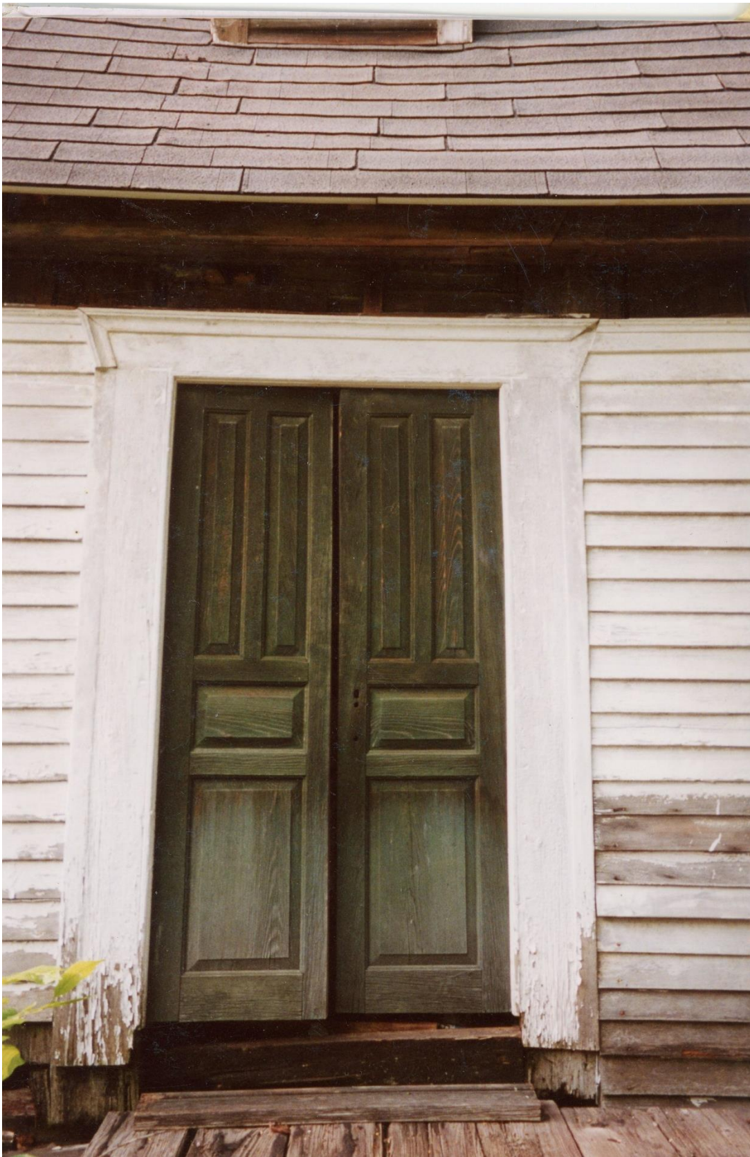
Figure C5b. Pre-Restoration, the Daniel Rose House 1741, West Granville. ‘Bedford Settlement Door Surround’ with pilasters and angled lintel acting as a pointer, directing attention to the eight-panel double-leaf door that may symbolize the eight blessings of the Sermon on the Mount (Matthew 5:3-12). Camera facing north. Photo by Bill Phelon, June 2001.
