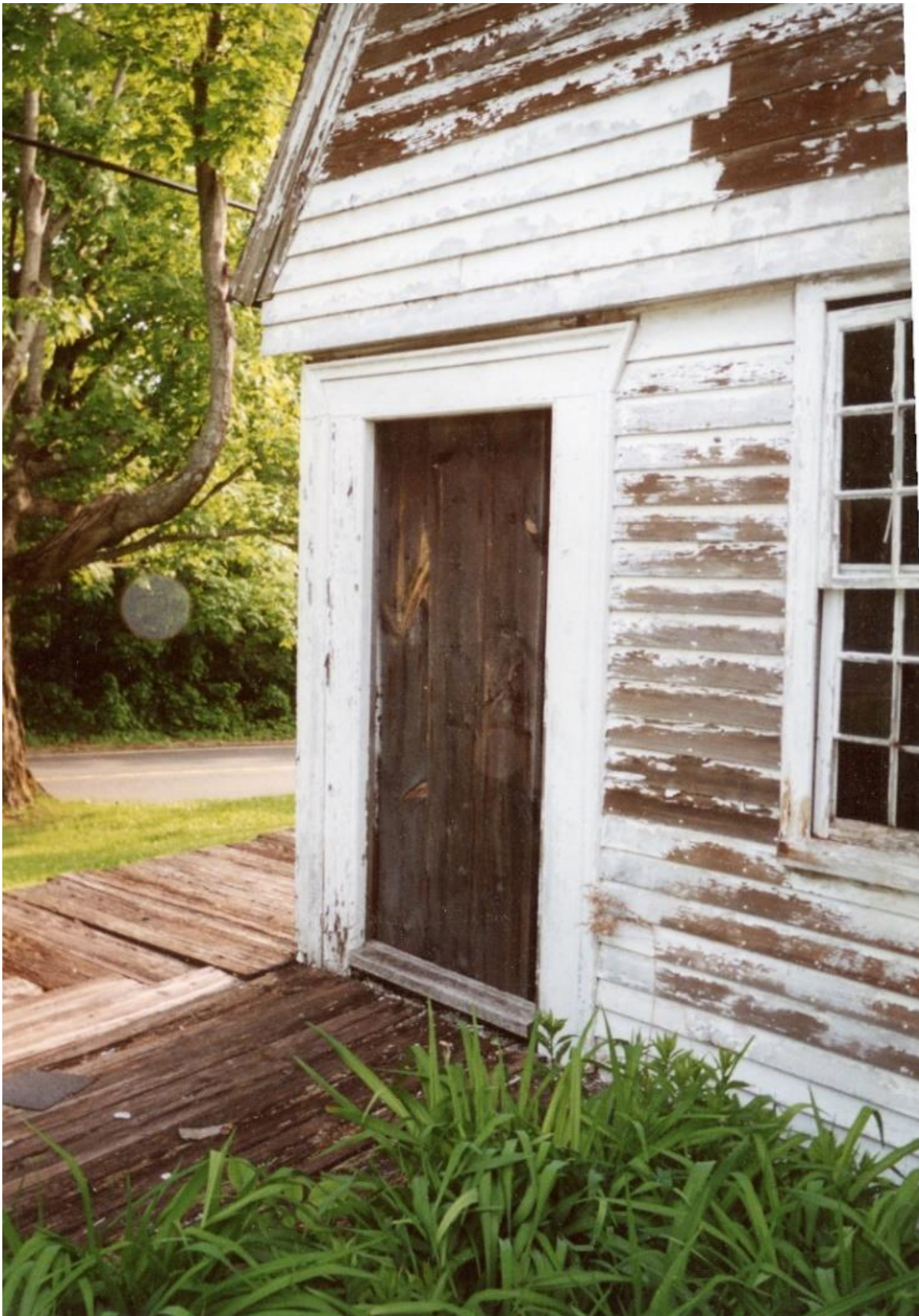
Figure C10. Pre-Restoration, the Daniel Rose House 1741, ‘Bedford Settlement Door Surround’ with pilasters and angled lintel of the front entry, repeated for the east-facing coffin door. Camera facing southwest. Photo by Bill Phelon, June 2001.
