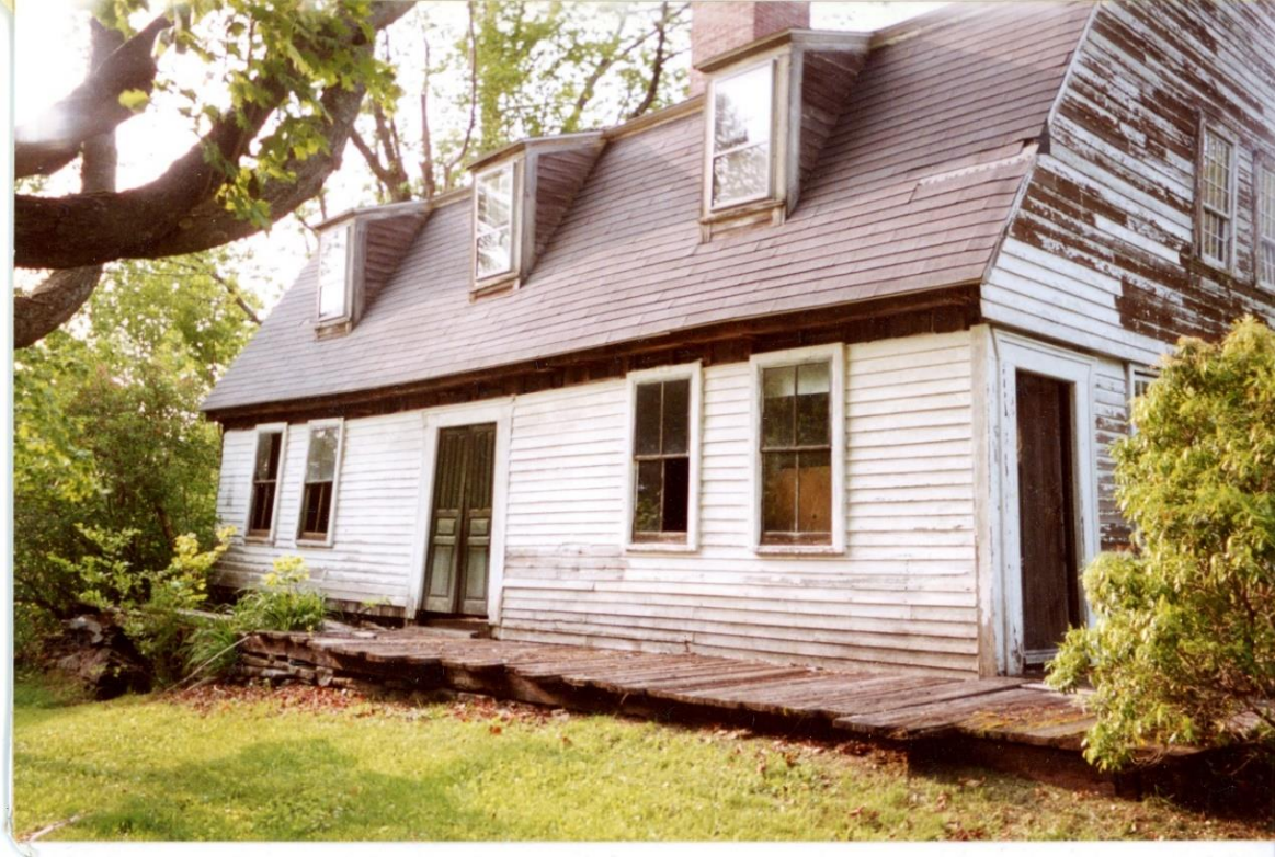
Figures C8. (Upper, Lower Left) Pre-Restoration, the Daniel Rose House 1741, Bedford Settlement Door Surrounds with pilasters and angled lintels at front entry and east-facing coffin door. Camera facing northwest. Figure C9. Interior view before craftsmanship of a reconstructed coffin door to replace original and restore clapboard siding. Camera facing east. Photos by Bill Phelon, June 2001. (Lower Right) Post-Restoration by Bill Phelon, Camera facing southeast, 2019.
