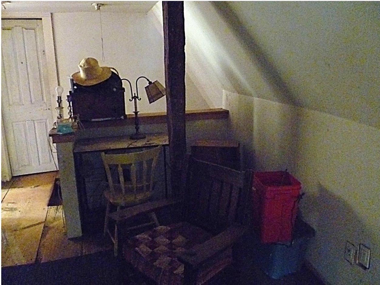
Figure 3.54. Interior structure is evident in unfinished landing at center of Daniel Rose House, second floor. Stairway beyond this partition leads down to the Keeping Room and this landing is also accessed from the north door of the Ballroom. Partly above the Keeping Room, this space would have been ideal for the storage of the “2 [spinning] wheels & 1 tape loom & 1 Old Chest, 3 [Bales] and \frac{3}{4} Sheeps wool” listed in Daniel Rose’s 1790 inventory. [This may have been the area in which Nelsie Harger Sheets was photographed ca. 1908 at work weaving on a large loom owned by her Aunt Eliza Harger Smith in the architecturally similar gambrel-roofed David Harger Place, once standing northwestward of the intersection of West Hartland Road and Main Road; and apparently, previously, owned by Charles Curtiss (until he moved to Ohio in 1811). David Harger boarded and lived with the Daniel Rose family during the American Revolution, as noted in his 1837 affidavit testifying to the (Castle Island) military service of Daniel’s son, Abner Rose when Abner’s widow Abigail Stebbins Rose filed for Abner’s Revolutionary War pension].
