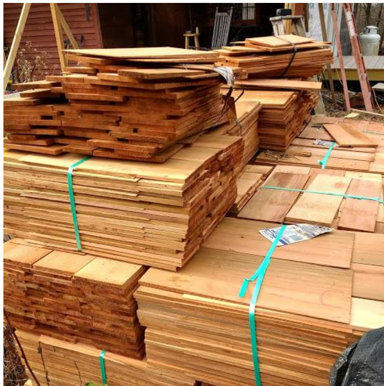
Figure 3.56b. In December 2017, a new roof was put on the two-story addition (ca. 1985) extending north from the keeping room, a potential ‘Docent Wing’: with Grace Ice and Water Shield underlayment, one layer of royal cedar breather and then two layers of red cedar perfection for “three sheets (of shingles) to the wind” in the old tradition. Camera facing west. Photos, December 2017.
