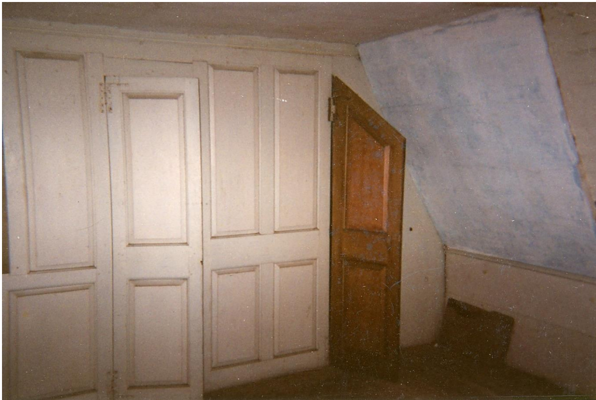
Figure 3.42. Daniel Rose House, Upstairs Southwest Bedchamber. According to the Legacy Inventory, 1985, the breast wall has “field raised panels.” (Upper) Breast wall, east. Camera facing east. (Lower) East Breast wall continued and south east front (gambrel) wall. Camera facing southeast. Painted panel door partially open to the left, accesses chimney stonework; natural wood color panel door to right accesses front stair landing. Photos, ca. July 2004.
