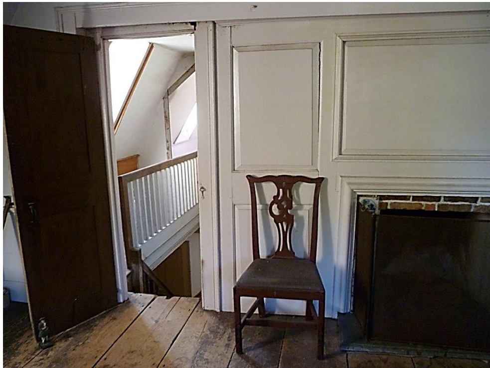
Figure 3.44. Front Southeast Bedchamber and Ballroom, second floor. (Upper) Sealed doorway in process of removal (see crowbar on chair) is first revealed here during restoration of chimney breast wall with fielded panels. The door to the upstairs hall landing and front stair entrance hall may have been sealed before or ca. 1813 when Lt. Jacob Baldwin's estate settlement apportioned the east half of the house (including the Ballroom) to his oldest son Heman and the west side to second oldest son Denizen. Cameras facing west. (Upper) Photo by Bill Phelon, ca. July 2004. (Lower) Photo, September 2019.
