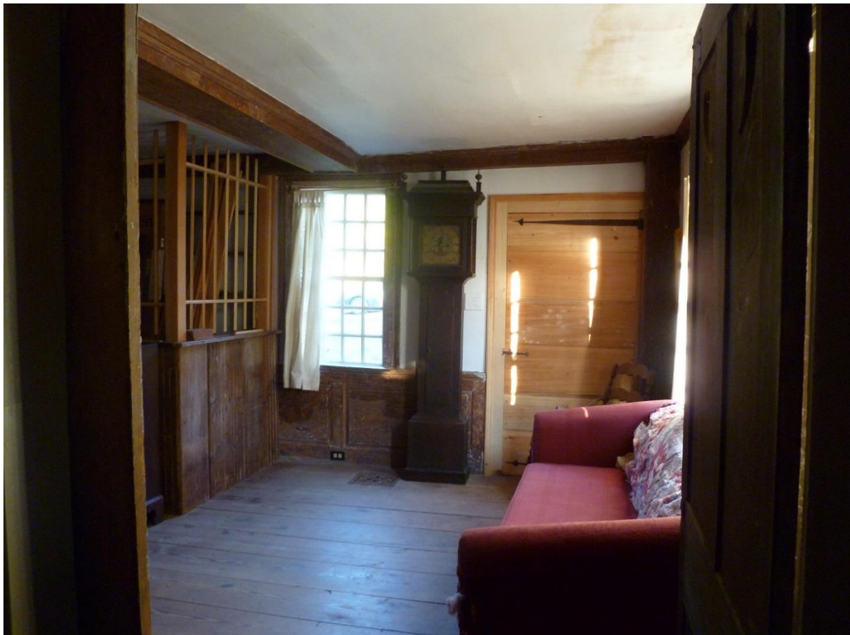
Figure 3.28. Daniel Rose House 1741. (Upper) Southeast Front Parlor (Tavern Room), interior view before restoration of original 12 over 12 front windows and repair of sashes throughout; craftsmanship of a reconstructed coffin door to replace original and restore entry clapboarding; reconstruction of original cage bar; hand removal of layers of paint from original woodwork of wainscot, corner post and summer beam with beading; and restoration of ceiling plaster. Heart door to right. Camera facing east, June 2001. (Lower) Paint removed from dado, corner post, summer beam, and flooring. Photo, September 2019.
