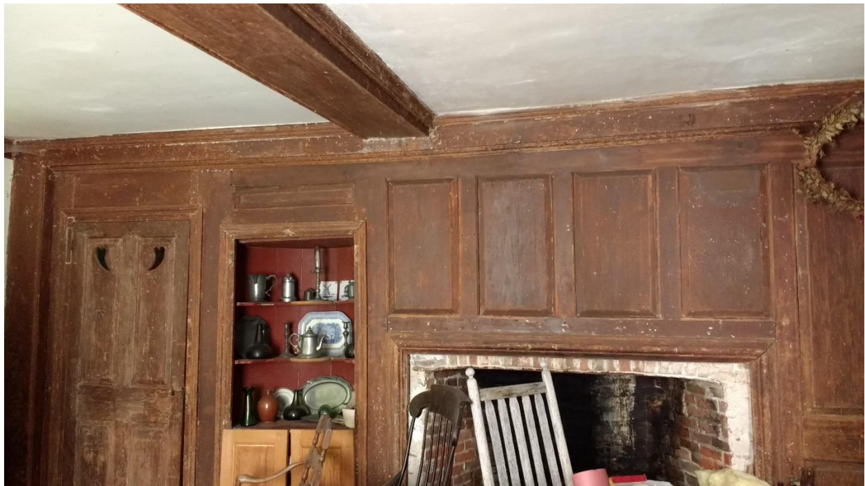
Figure 3.31. Tavern Room, Southeast Front Parlor, Daniel Rose House 1741. (Upper) Photo unlabeled, believed to be Tavern Room beam with breast wall removed to reveal chimney. Photo, July 2004. (Lower) Original wood surfaces of chimney breast wall with raised panels, encased chamfered and beaded summer beam and corner post restored by Bill Phelon. Original wood surfaces, flooring restored. Hearts in shape of powder horns are carved in the door of this home to six Revolutionary War veterans. Artilleryman Abner Rose and his wife Abigail Stebbins Rose were married in her birthplace, Springfield, MA, on February 8, 1781 (intentions published October 28, 1780) during the American Revolution and according to Abigail, “they removed immediately to Granville and lived in the family of his Father.” Camera facing west. August 2017.
