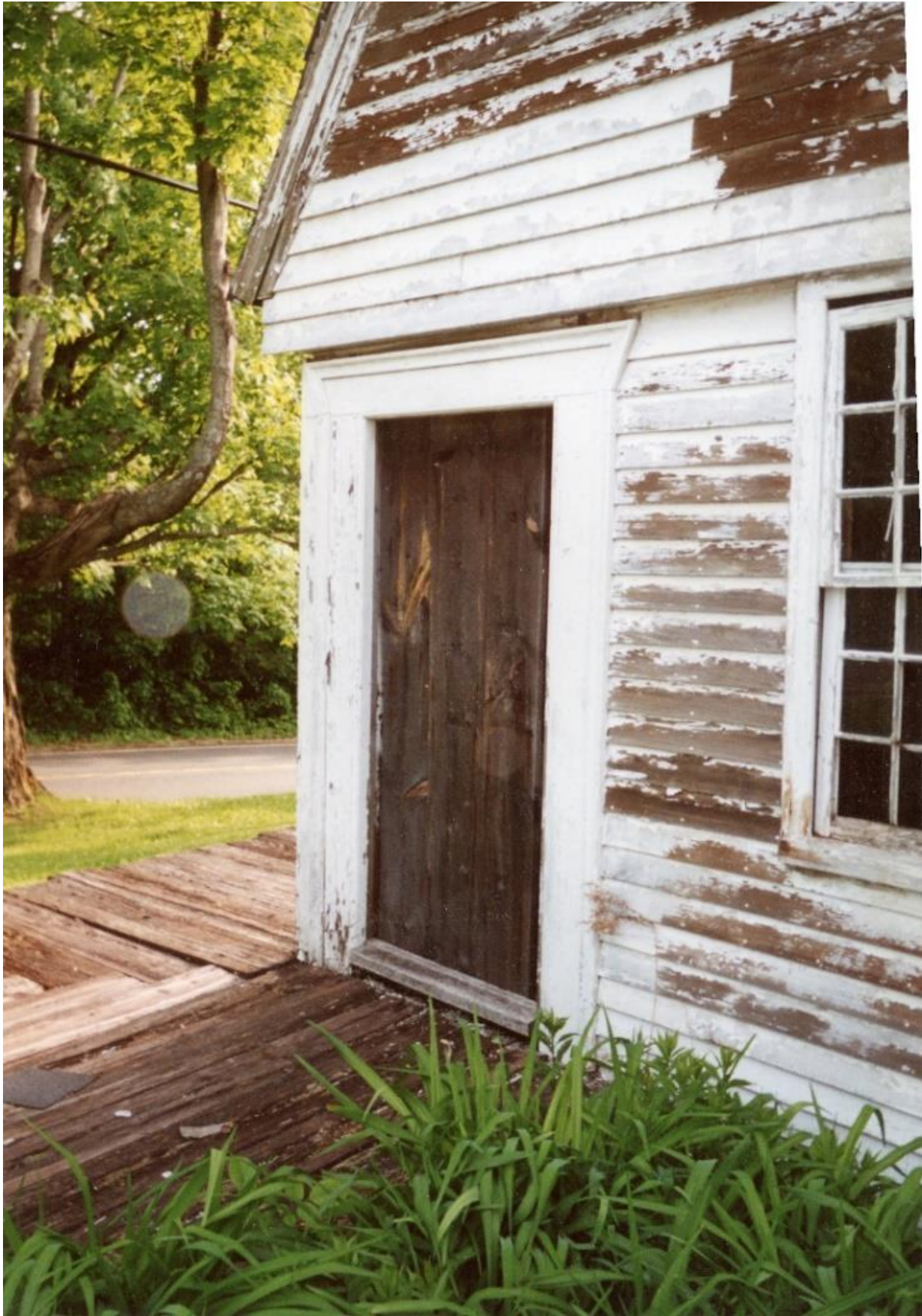
Figure 3.7. The Daniel Rose House, 1741, 'Bedford Settlement Door Surround' with the pilasters and angled lintel of the front entry, repeated for this east facing 'coffin door'. Camera facing southwest, June 2001.
