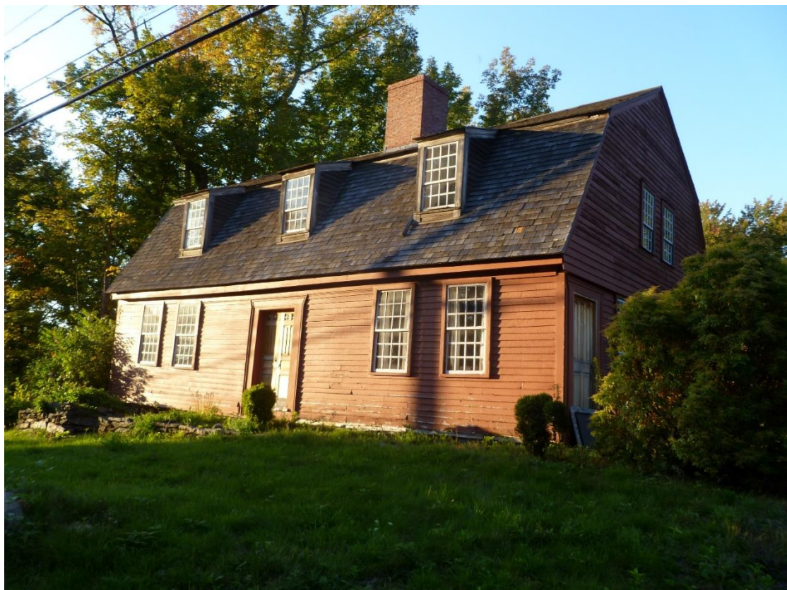
Figure 3.6. Daniel Rose House, 1741. (Upper) Camera facing northwest, June 2001. (Lower) After restoration by Bill Phelon, September 2019.
