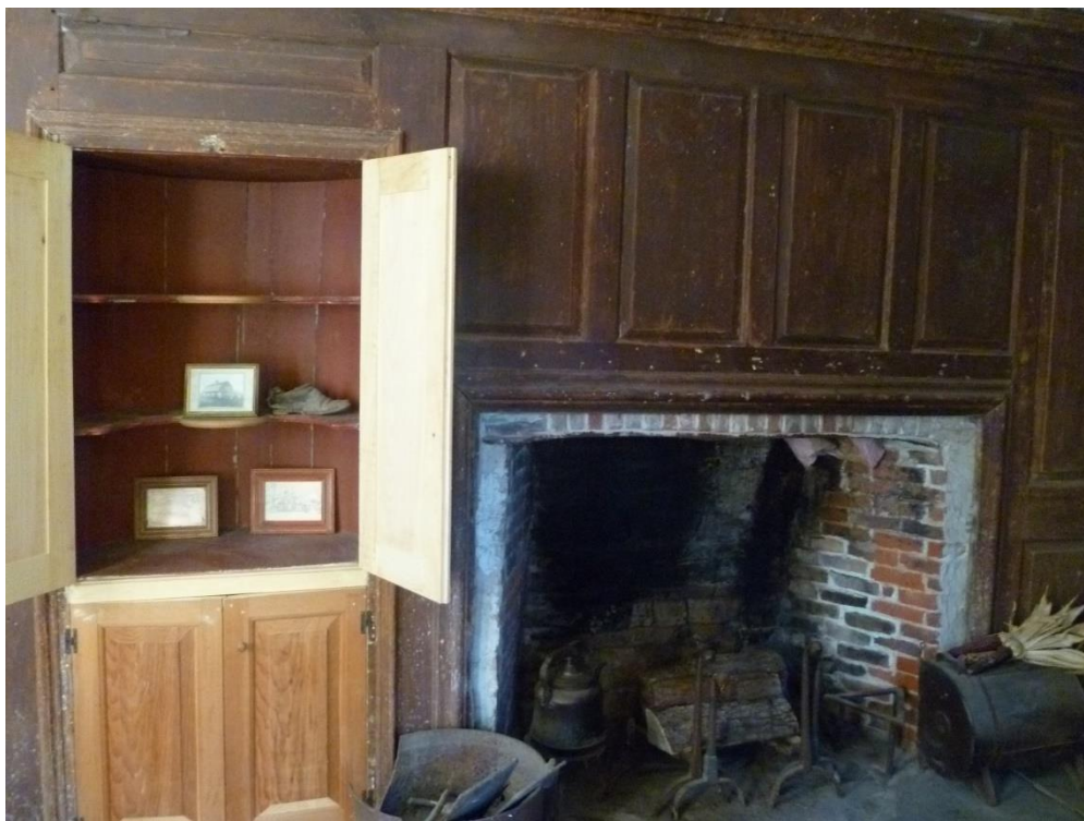
Figure 3.33. Southeast Front Parlor and Tavern Room, wood floor, summer beam, and chimney breast wall with raised panels was restored with old layers of paint removed by Bill Phelon. Cupboard doors were reconstructed, with old hinge marks still extant for proportion. Front hall is through door to the left (upper photo). The Legacy Inventory of 1985 documented the “floor to ceiling wall cupboard with scalloped shelves on upper half.” Camera facing west. Photos, September 2019.
