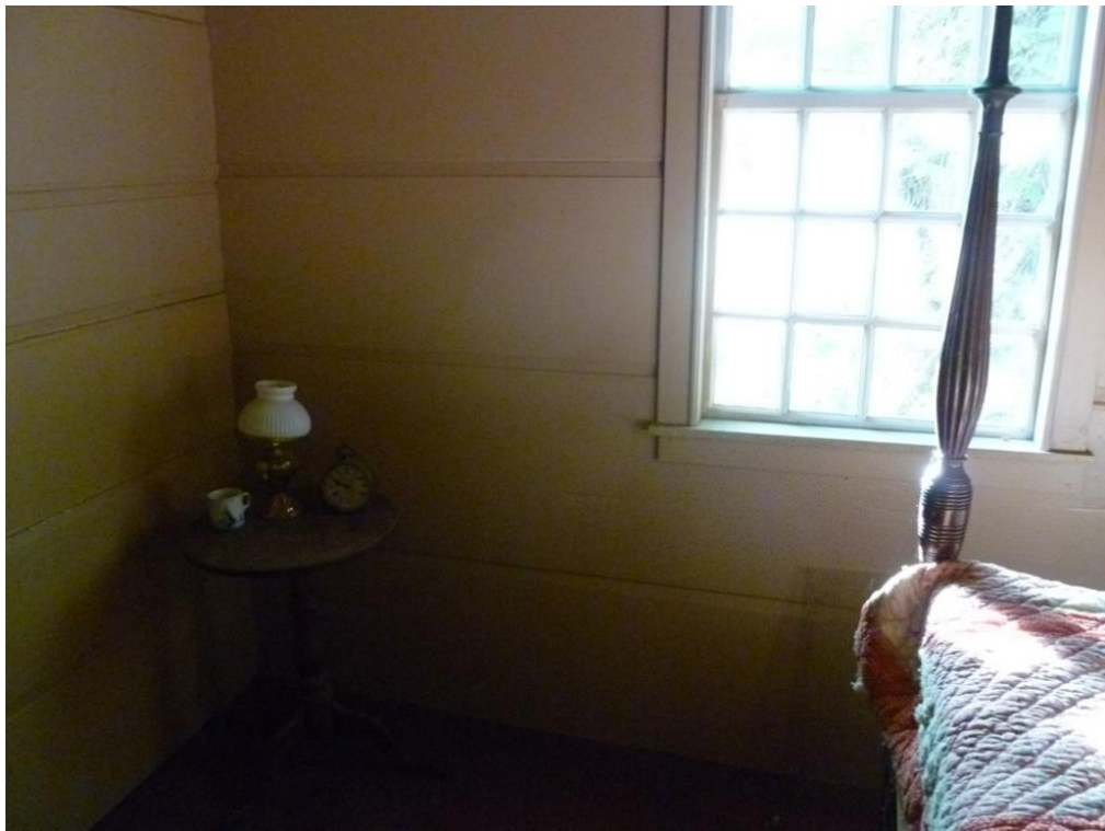
Figure 3.37. Achsah, known as ‘Achsy’ Rose gave birth to eleven children, seven born during the French and Indian Wars, in this Boring Room located west, off the Keeping Room. Horizontal pine sheathing on three walls, seen here (Upper) on west wall and (Lower) at southwest corner walls. The horizontal feather edge pine sheathing that was unpainted in 1985, required extensive restoration and painting. According to the Legacy Inventory of 1985, the original flooring remains. Photos, Sept. 2019. The quilt tradition in this room dates to the Olive Curtiss Baker quilt made in Granville in 1798; it was owned in this house by Olive’s son, Francis Graves Baker and given by his daughter, Laura who grew up in this house, to the Pocumtuck Valley Memorial Association before 1886 when the quilt was exhibited in Deerfield at Memorial Hall Museum where it is now.
