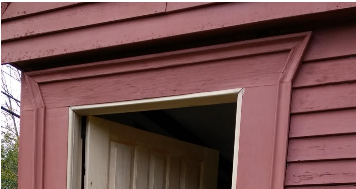
Figure 3.8. Daniel Rose House, 1741. Upstairs Ballroom windows of ‘12 over 8’ panes repeat number ‘8’ of the eight-paneled double-leaf front entry door, suggesting eight blessings of the Sermon on the Mount as found in western church architecture. East façade, camera facing west, June 2001. (Lower) Original architrave, herein called the ‘Bedford Settlement Door Surround’ for east facing door, is of the same detail as the front architrave with pilasters and angled lintel. Reconstructed coffin door reproduces the door seen in Fig. 3.10, the Kitchen Garden photo of 2017 (not the vertical plank door in Fig. 3.7). Camera facing southwest. Photo, October 2017.
