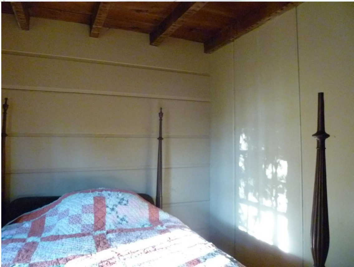
Figure 3.35. Borning Room located west off the Keeping Room. Horizontal (north wall to left and vertical (east wall to right) feather edge pine sheathing and smooth planed sub flooring visible overhead, as mentioned in the 2003 Curtis report at the Granville Public Library Historical Room. (Upper) Photo during restoration, 2004. Camera facing northeast. (Lower) Photo, September 2019.
