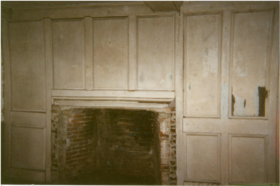
Figure 3.38. Southwest Front Parlor, Daniel Rose House. Color analysis on one panel to the right indicated original green paint, as also found in the front hallway (Fig. 3.41). This paint color is reminiscent of the green dyed wool quilt (now at Historic Deerfield, MA) made by Olive Curtiss Baker in 1798 and owned by her son Francis G. Baker at this house before, during and after the Civil War – the quilt inspired the Deerfield Arts and Crafts Movement. According to Legacy Inventory, 1985, the “Parlor Fireplace breast wall is field with bolection molding around fireplace opening. Perimeter is covered with wood panel dado plaster above. Ceiling beams, summer beams and corner post are cased and molded. Floors are wide pine boards original.” (Upper) Camera facing southeast. (Lower) Camera facing east, 2004.
