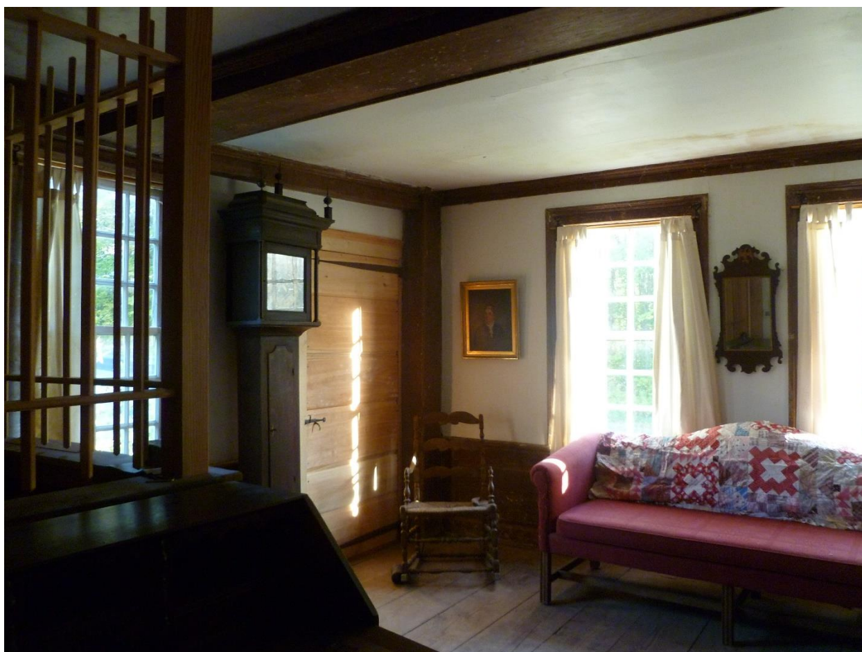
Figure 3.29. Southeast Front Parlor and Tavern Room, Daniel Rose House, 1741. Corner post and summer beam cased and molded and paneled dado with plaster above were restored by Bill Phelon with layers of paint removed. The Cage Bar reconstructed to meet specs of structural evidence of enclosure and shelves in the wainscot and walls and the east coffin door reconstruction were completed by Bob Bettcher, 18 th century Reconstructions and Restorations, 2017 as per Bill Phelon’s direction. Photo, September 2019, Camera facing southeast. The tradition of quilts in this house dates to the green dyed wool quilt with “elaborate patterns” (now at Historic Deerfield, MA) made in 1798 by Olive Curtiss Baker, wife of Rev. Joel Baker pastor for thirty-six years of the Second Church of Christ Congregational. Olive’s quilt was owned by her son Francis G. Baker at this house before, during and after the Civil War. Francis’ daughter Laura, who grew up in the Daniel Rose House, gave her grandmother’s quilt to the Pocumtuck Valley Memorial Association before 1886 when it was exhibited in the PVMA’s Memorial Hall Museum that year, in the first museum installation of a period bedroom in the United States, possibly the world. The Baker quilt inspired the Deerfield Arts and Crafts Movement in 1896 and is now owned by the Pocumtuck Valley Memorial Association at Old Deerfield.
