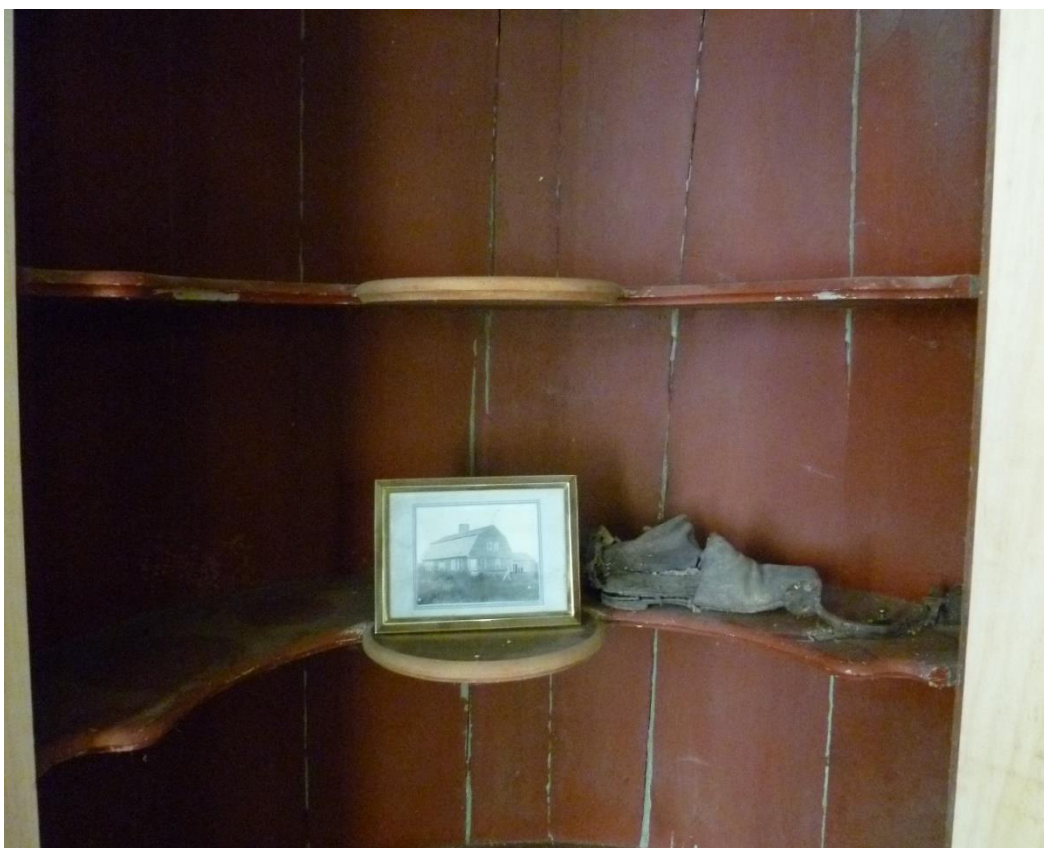
Figure 3.34. Southeast Front Parlor and Tavern Room, Daniel Rose House, restored cupboard in chimney breast wall. Camera facing west. Photo, September 2019.
