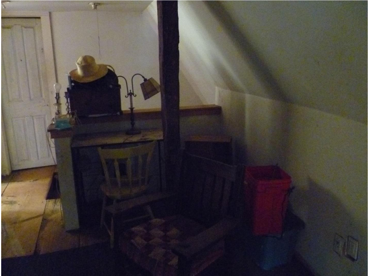
Figure 69. Interior structure is evident in unfinished landing at center of house, second floor, Daniel Rose House. The following Bedchamber is to the left. Stairway beyond this partition leads down to Keeping Room. Hallway to potential Docent Wing with second floor bath and bedroom is behind the camera. Camera facing west.
