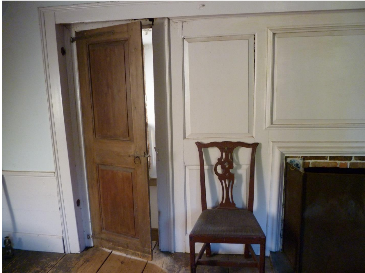
Figure 63. Front Southeast Bedchamber and Ballroom chimney breastwall with fielded panels, Daniel Rose House. Stairway and landing are through the doorway. Camera facing southwest.
