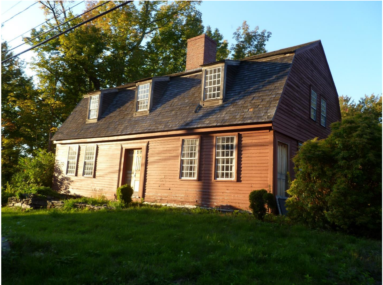
Figures 74. Daniel Rose House, West Granville National Register Historic District. Perspective view, camera facing northwest. September 2019.
