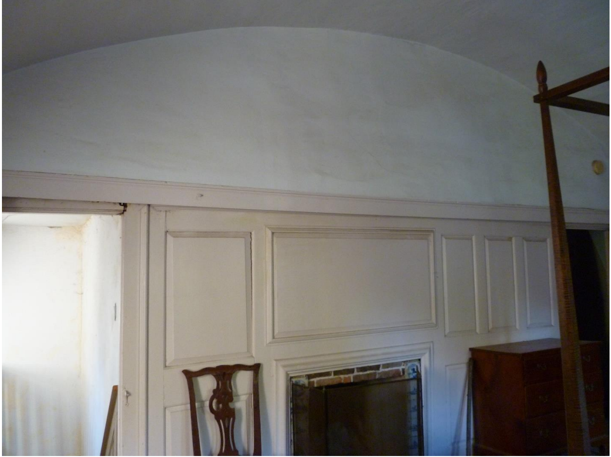
Figure 67. Front Southeast Bedchamber vaulted ceiling twelve feet high and chimney breastwall with raised panels, Daniel Rose House. View to Stairway and landing at front entryway. Camera facing west.
