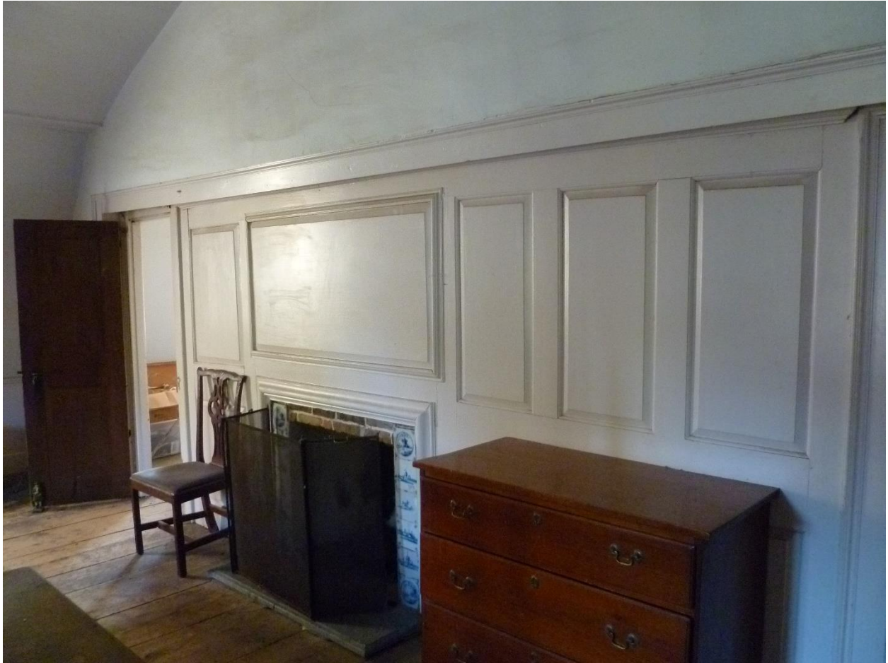
Figure 66. Front Southeast Bedchamber chimney breastwall with fielded panels restored by Bill Phelon, Daniel Rose House. During restoration, there was evidence of blue paint on remaining original wall-to-ceiling plaster. View to Stairway and landing at front entryway. Camera facing southwest.
