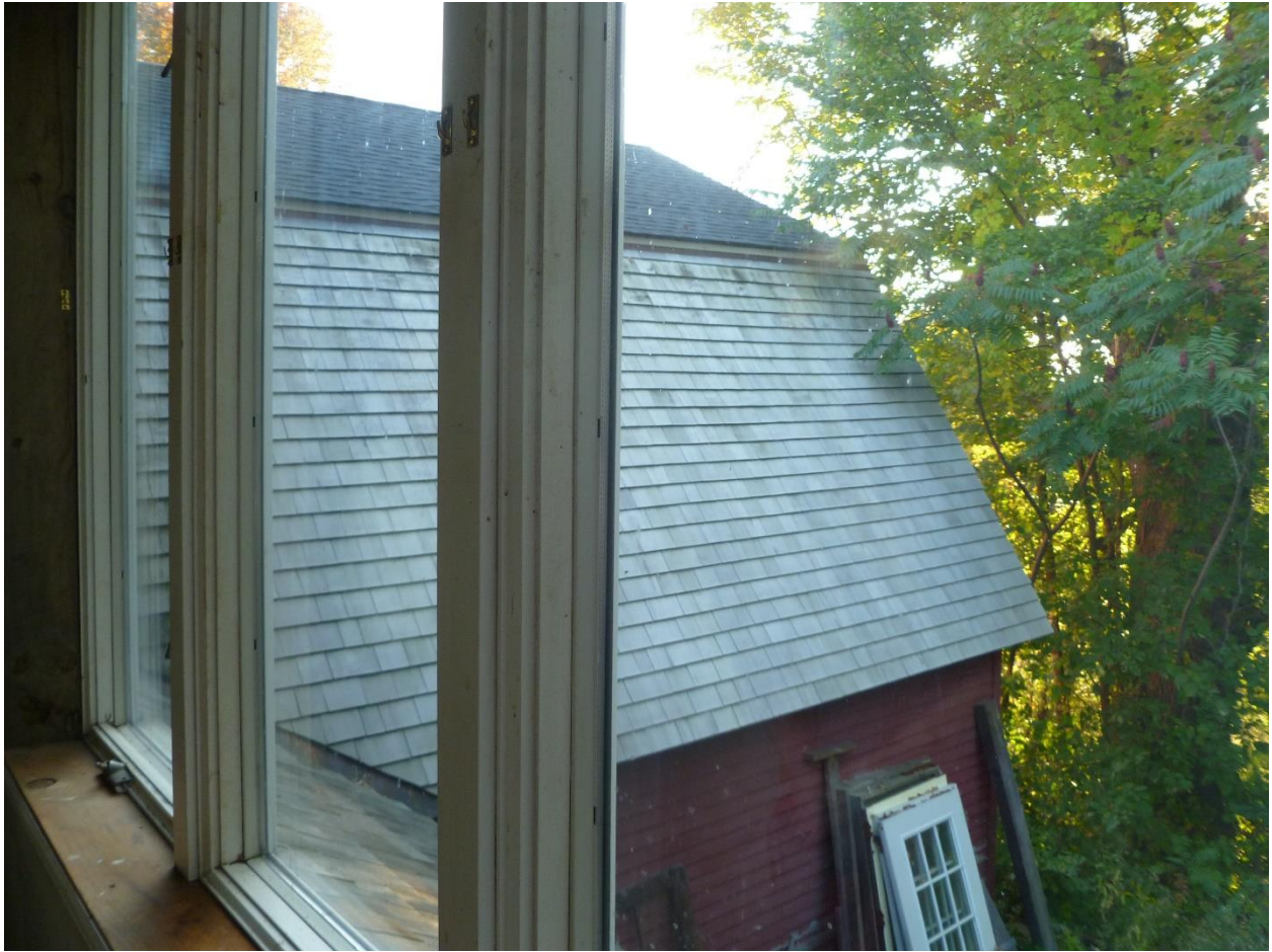
Figures 71. View of western side of main house from second floor hall updated windows of the potential Docent Wing two-story extension ca. 1900, 1930 housing upstairs bath and bedroom; and downstairs kitchen and sitting room. Camera facing southwest. September 2019.
