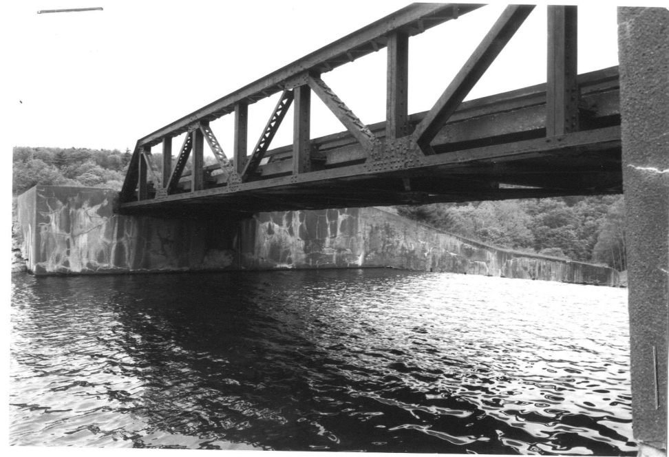
W TRUSS FROM SW
