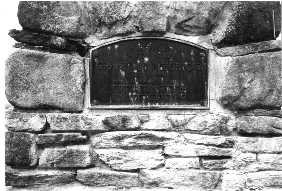
INS END POST, SE APPROACH WALL
