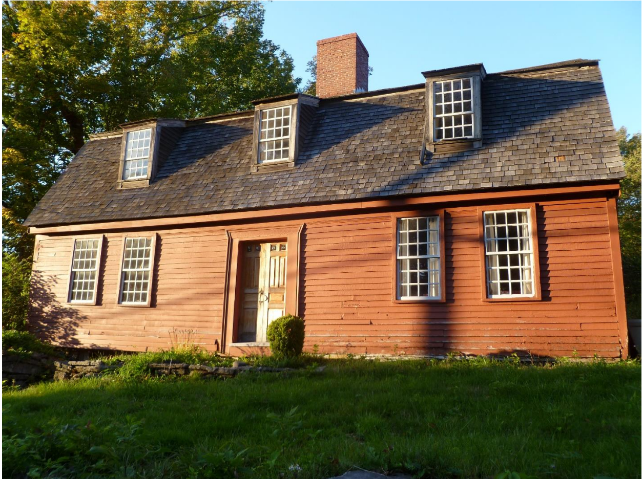
Figure 6: Daniel Rose House with structural evidence of fortification in the front façade. According to William Brian Phelon (2013), “In the westward facing foundation wall there are what appear to be two cannon ports each 15” wide and 10” high with a bottom sill 30” off the ground. Other evidence like a gun port over the front door, a level foundation wall across the front of the house to support a pallisade, mortices in the front surface of the front posts (with pieces of broken off tenons and trunnels) and framing modifications to enclose a well support the theory this was a fort.”
