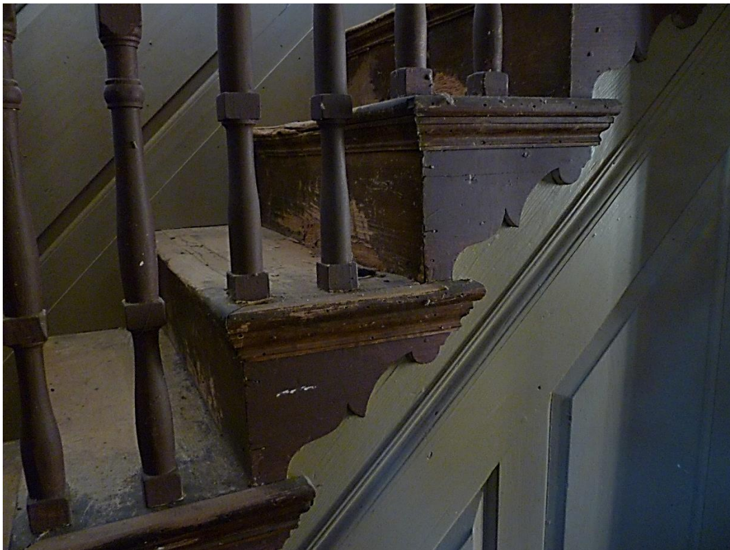
48. Perhaps an indication of the green dye used for Olive Curtiss Baker's whole-cloth quilt, the green paint color found in the front southwest parlor, was restored on the raised panels of this Front Hall staircase with details. Stair risers and treads appropriately rose to the east. The Daniel Rose-Baldwin-Baker-Phelon House, 1741.
