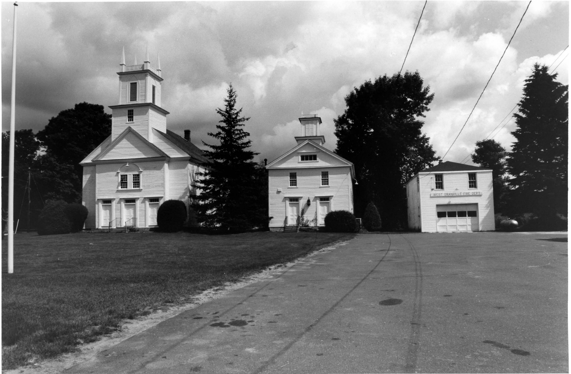
1- View of the West Granville Church, GRN.16; the West Granville Academy, GRN.17; and the West Granville Fire Station (nc).
