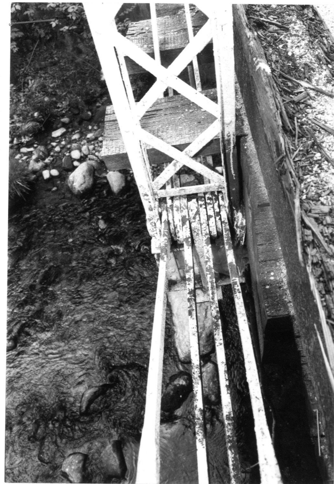
CENTER VERTICAL, LOWER PANEL POINT, N TRUSS (5-16-85)
