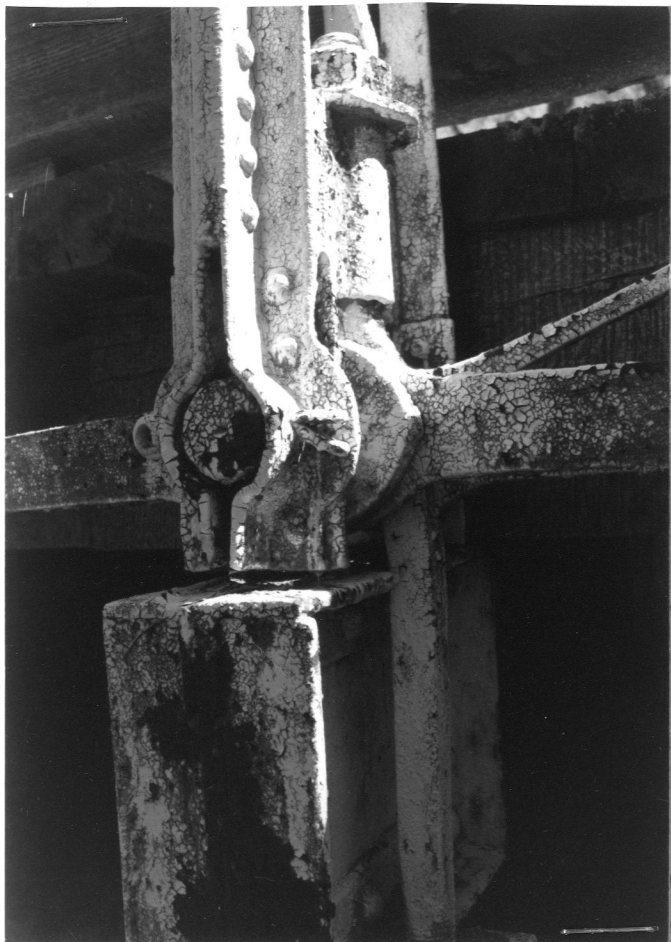
S TRUSS, W VERTICAL LOWER END, FROM SW (5-4-85)
