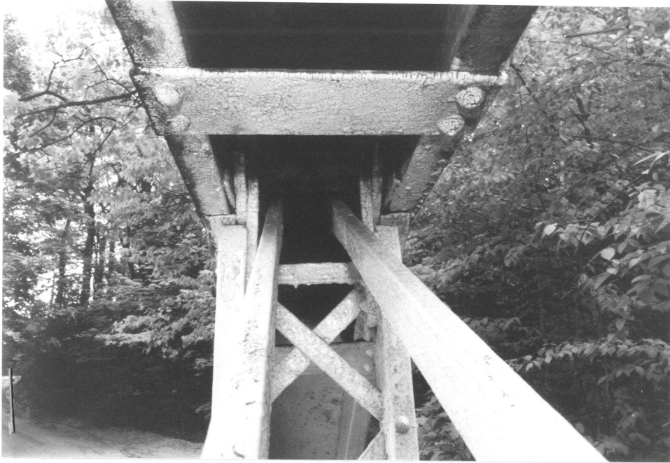
S TRUSS, E END, 1ST UPPER PANEL POINT
