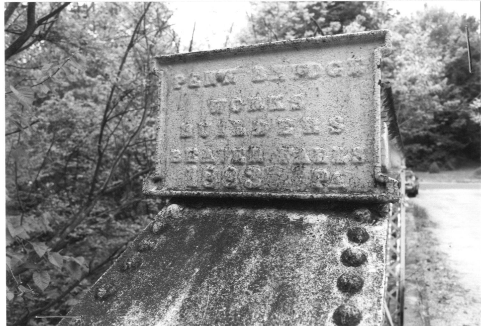
ON E END, UPPER CHORD, S TRUSS
