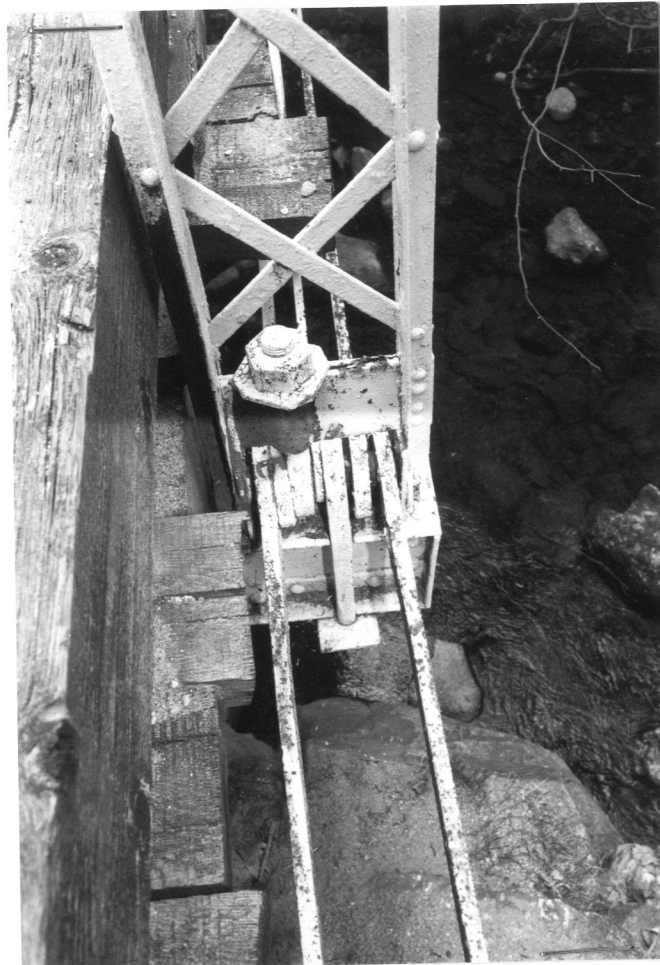
END VERTICAL, LOWER PANEL POINT, LOOKING TOWARD CENTER PANELS, S TRUSS (5-16-85)
