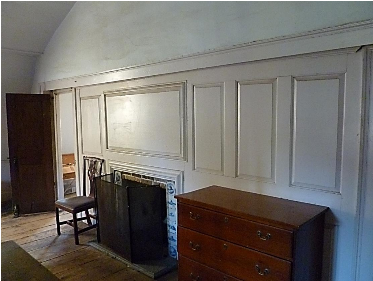
Ballroom, west breast wall. This Southeast Bed Chamber runs the entire width of the Daniel Rose House, with the barrel-vaulted ceiling rising to a height of twelve feet. There is evidence of benches along the window wall. Camera facing southwest. Photograph, 2019.
