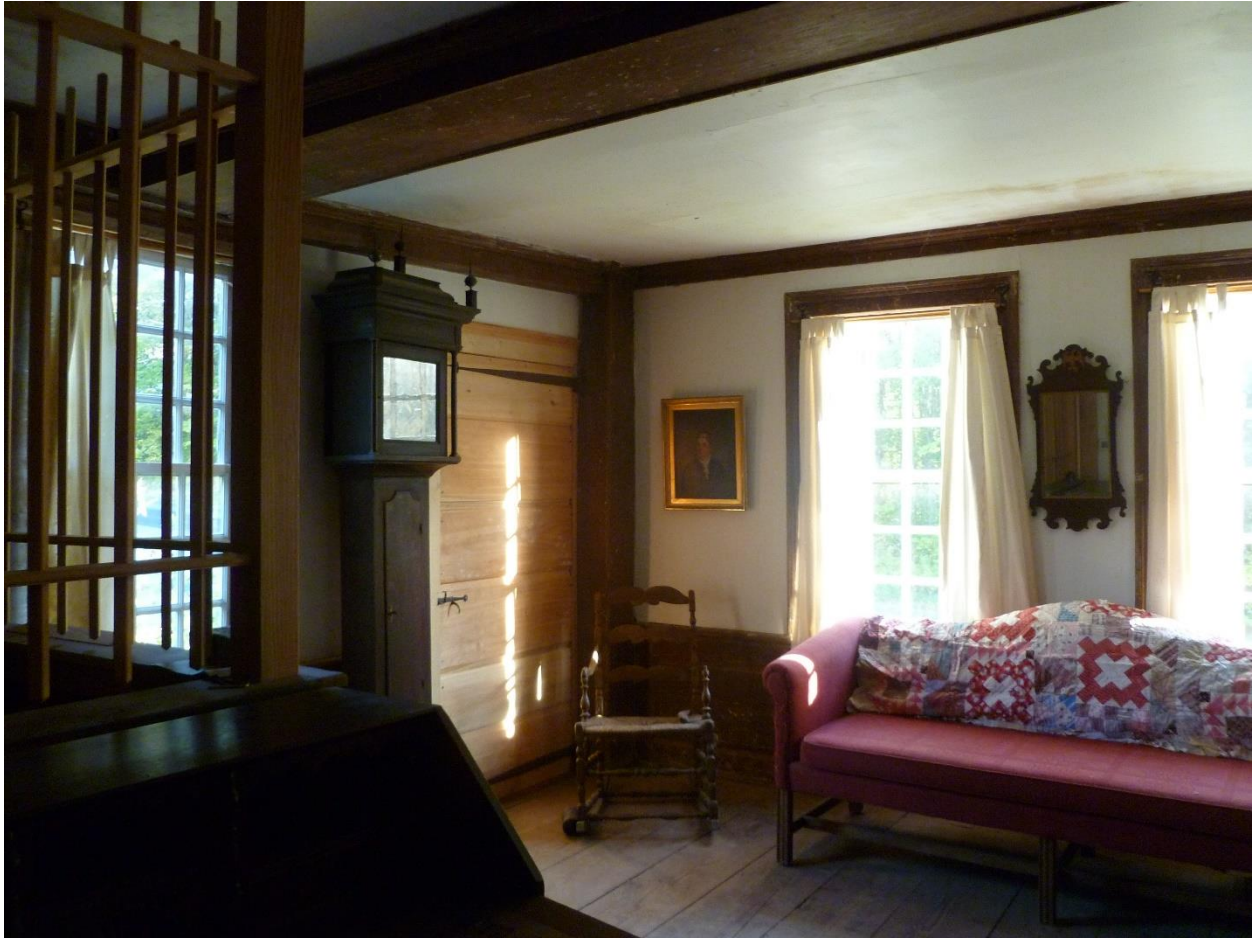
Figure 41. Southeast Front Parlor and Tavern Room, Daniel Rose House. Corner post and summer beam cased and molded and paneled dado with plaster above were restored by Bill Phelon. The Cage Bar reconstructed to meet specs of structural evidence of enclosure and shelves in the wainscot and walls and the east Coffin Door reconstruction were completed by Bob Bettcher, 18 th century Reconstructions and Restorations, 2017. Camera facing southeast.
