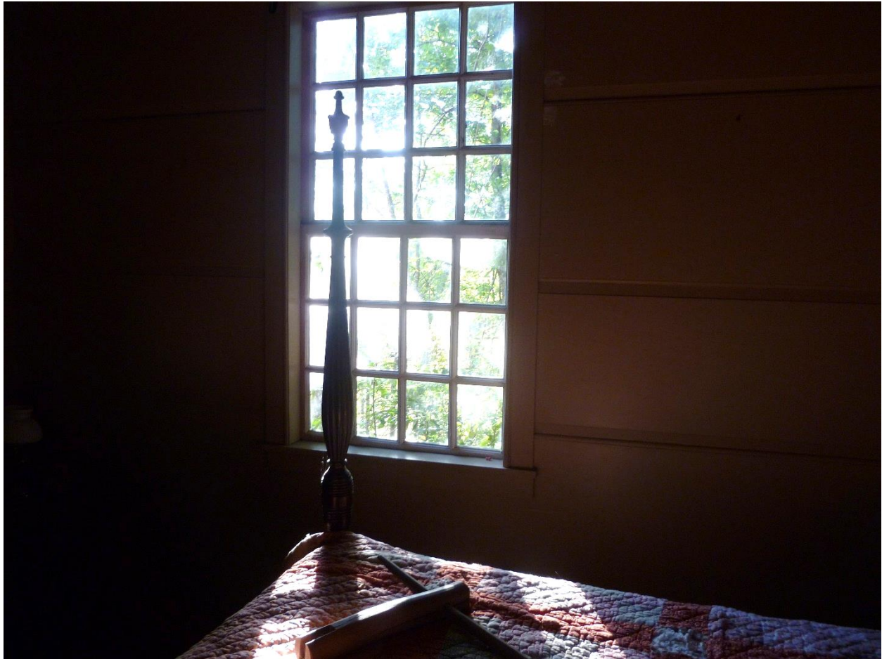
Figures 50-51. The Borning room located west off the Keeping Room, Daniel Rose House. Horizontal pine sheathing restored by Bill Phelon. Camera facing west with a view of the landscape below. September 2019. This room is above the west cellar wall with ports for gun mounts.
