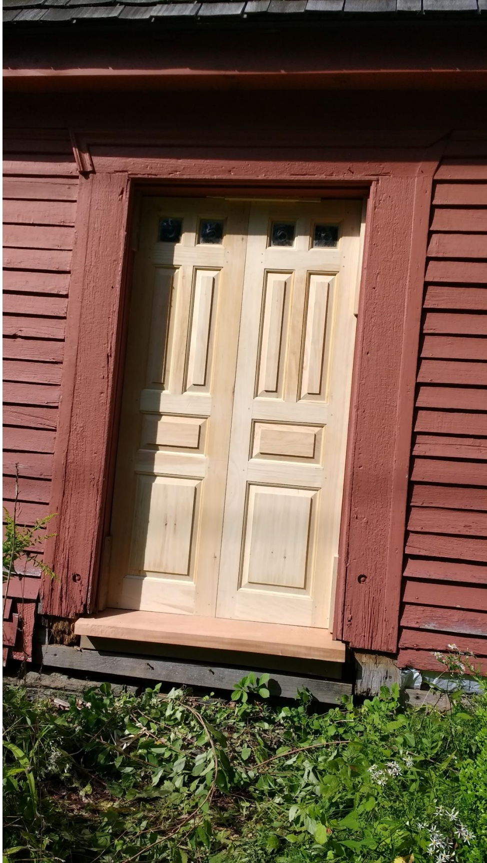
Figures 31. Reconstructed front double-leaf door with bull's eye glass added, Daniel Rose House. Camera facing southwest. October 2017. The center entry features the original "simple architrave" according to the West Granville National Register Historic District Form, 1991, Sect.7.5.
