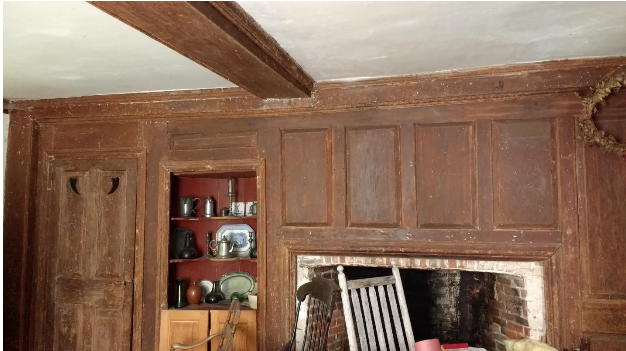
Figure 42. Southeast Front Parlor Chimney breastwall and encased chamfered and beaded summer beam restored by Bill Phelon. Note hearts in shape of powder horns in door. This was home to six Revolutionary War veterans. Abner Rose and his wife Abigail Stebbins Rose were married in her birthplace, Springfield, MA, on February 8, 1781 (intentions published October 28, 1780) during the American Revolution and according to Abigail, “they removed immediately to Granville and lived in the family of his Father.” Camera facing west. August 2017.
