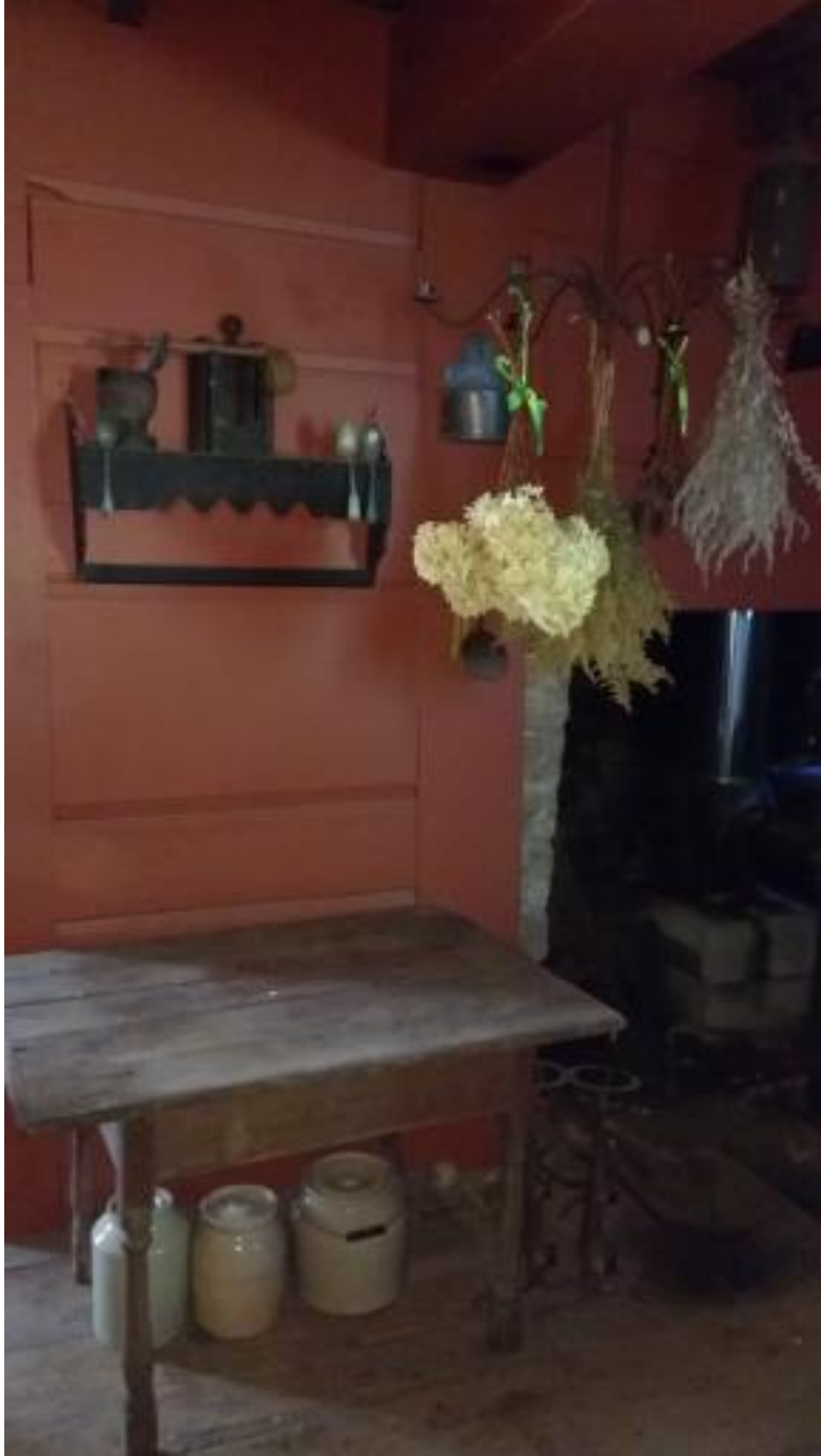
Figure 36. Keeping Room breastwall with feather edge pine panels and open beam, north to south. Camera facing southwest. August 2017.
