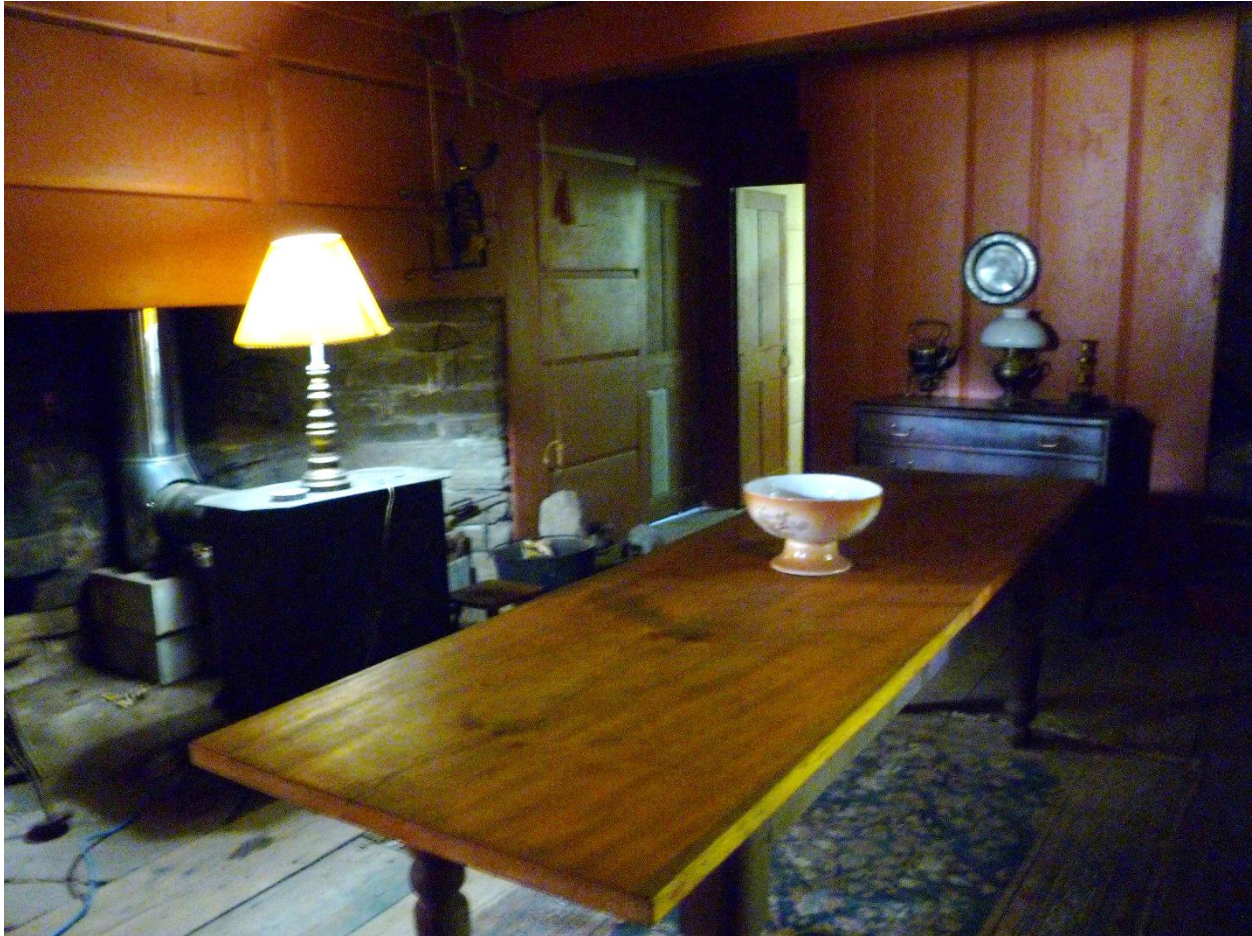
Figure 33. Keeping Room Hearth. According to Curtis, March 24, 2003: “A stone chimney base and stack are features more commonly seen in Connecticut contexts and then, generally seen no later than the third quarter of the 18 th century. Fire boxes are deep and straight sided; certainly not the Rumford configuration that becomes so prevalent at the end of the 18 th century. The cavernous kitchen fireplace, with its stone firebox, bake oven situated at the rear, and provision for lug poles to be suspended within the flu, is a throw-back to the early 18 th century.”
