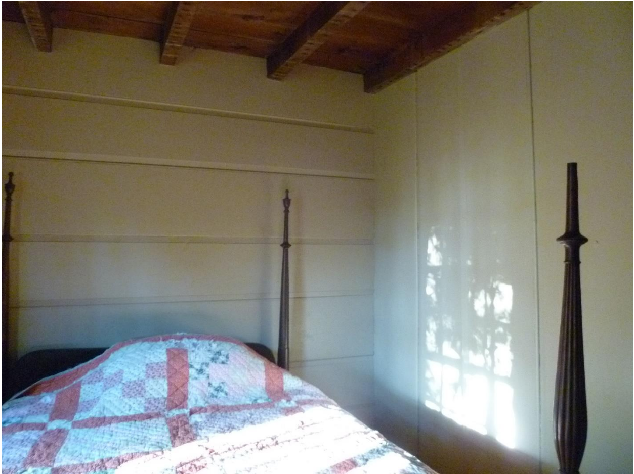
Figure 53. Bedding room located west off the Keeping room. Note the horizontal (north wall to left and vertical (east wall to right) feather edge pine sheathing and smooth planed sub flooring visible overhead, as mentioned in the 2003 Curtis report at the Granville Public Library Historical Room. Camera facing northeast. September 2019.
