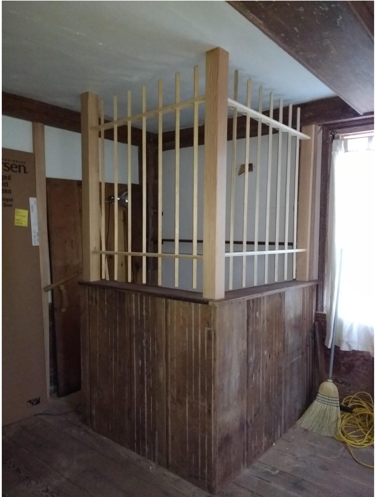
Figure 48. Southeast Front Parlor and Tap Room with reconstructed Cage Bar to meet specs of structural evidence including notches in the wainscot. Cage Bar reconstructed by Bob Bettcher, 18 th century Reconstructions and Restorations, 2017. Camera facing northeast, near where the Shoe (see below) was discovered in the wall. August 2017.
