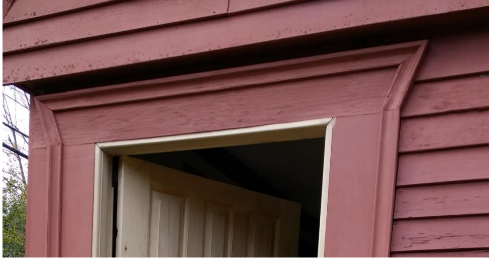
Figure 32. Original architrave, east coffin door is of the same detail as the front architrave, described as a “simple architrave” in the West Granville National Register Historic District Form, 1991, Sect.7.5. Daniel Rose House. Camera facing southwest. October 2017.
