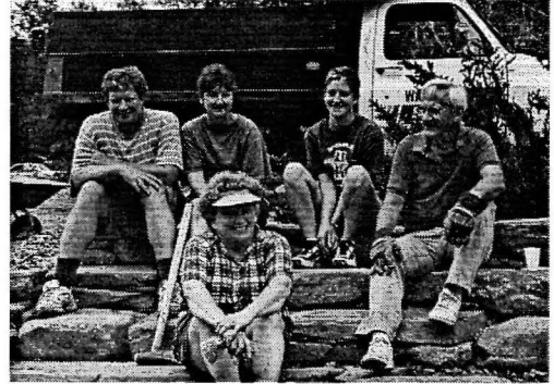
Part of the wall building team.
