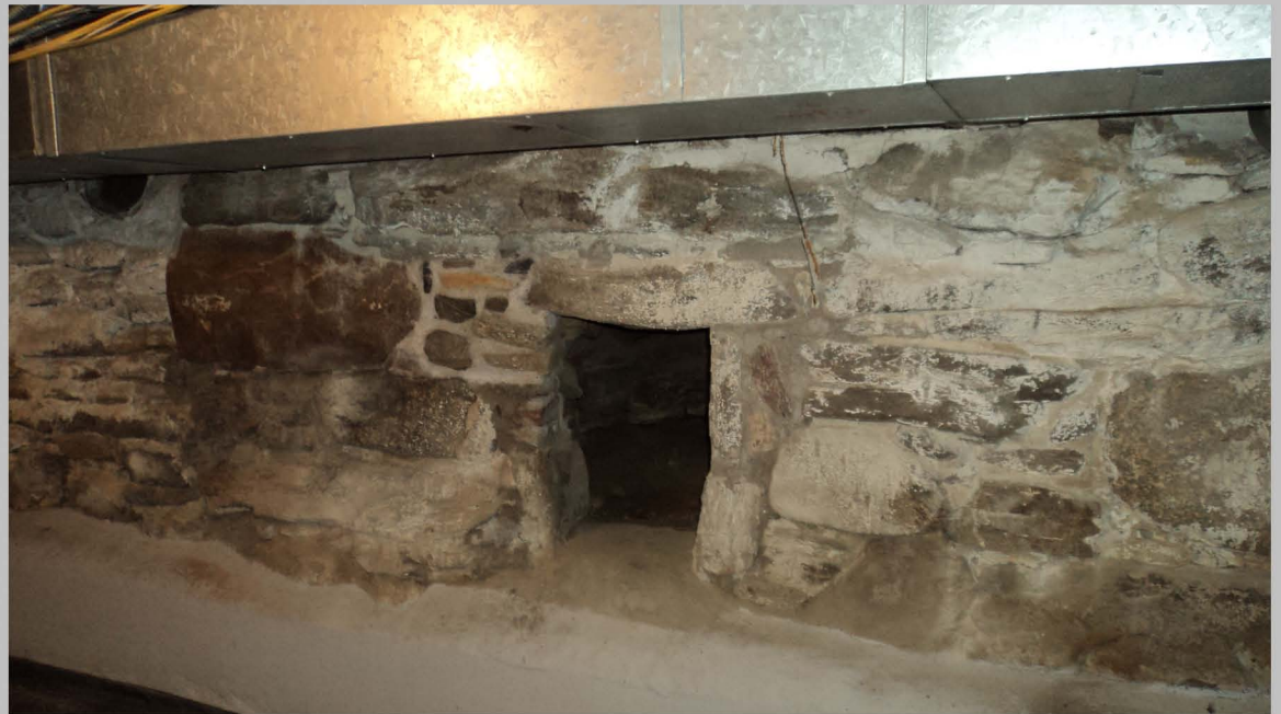
26. Main block, chimney foundation, view to southwest.
