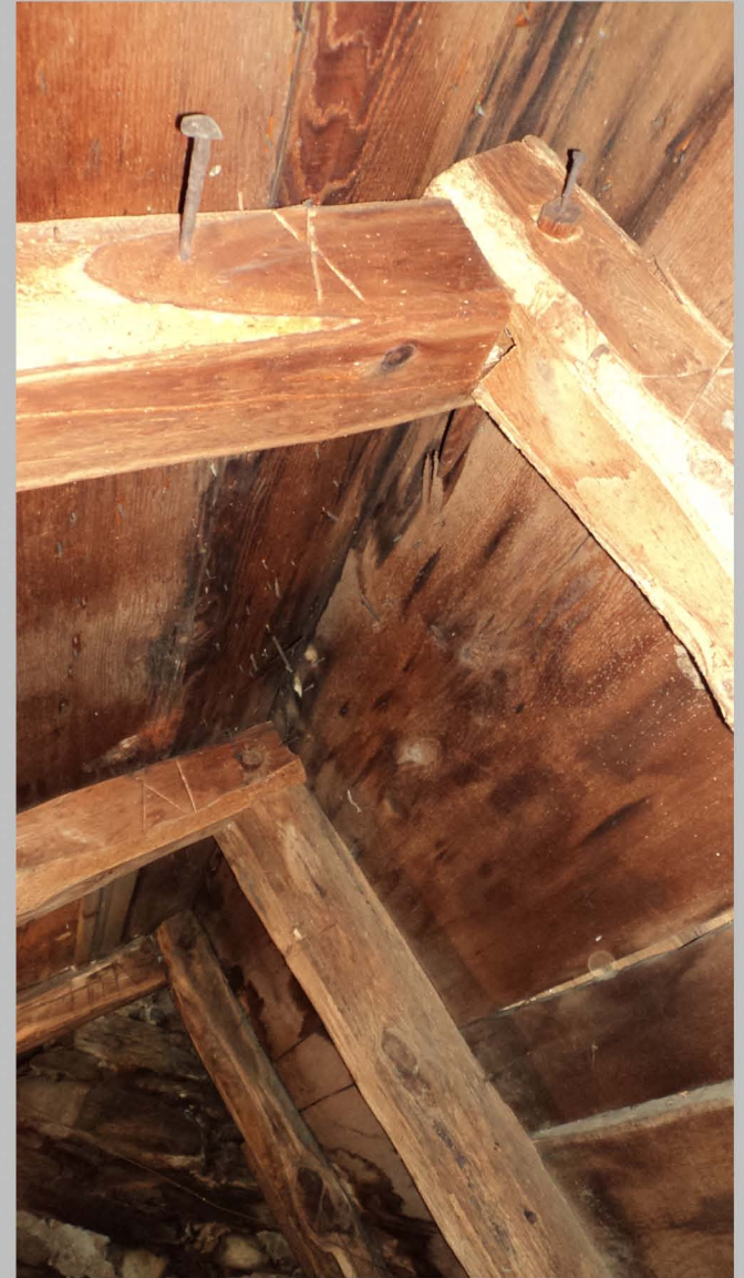
20. Scribe rule markings, attic main block, view to west.
