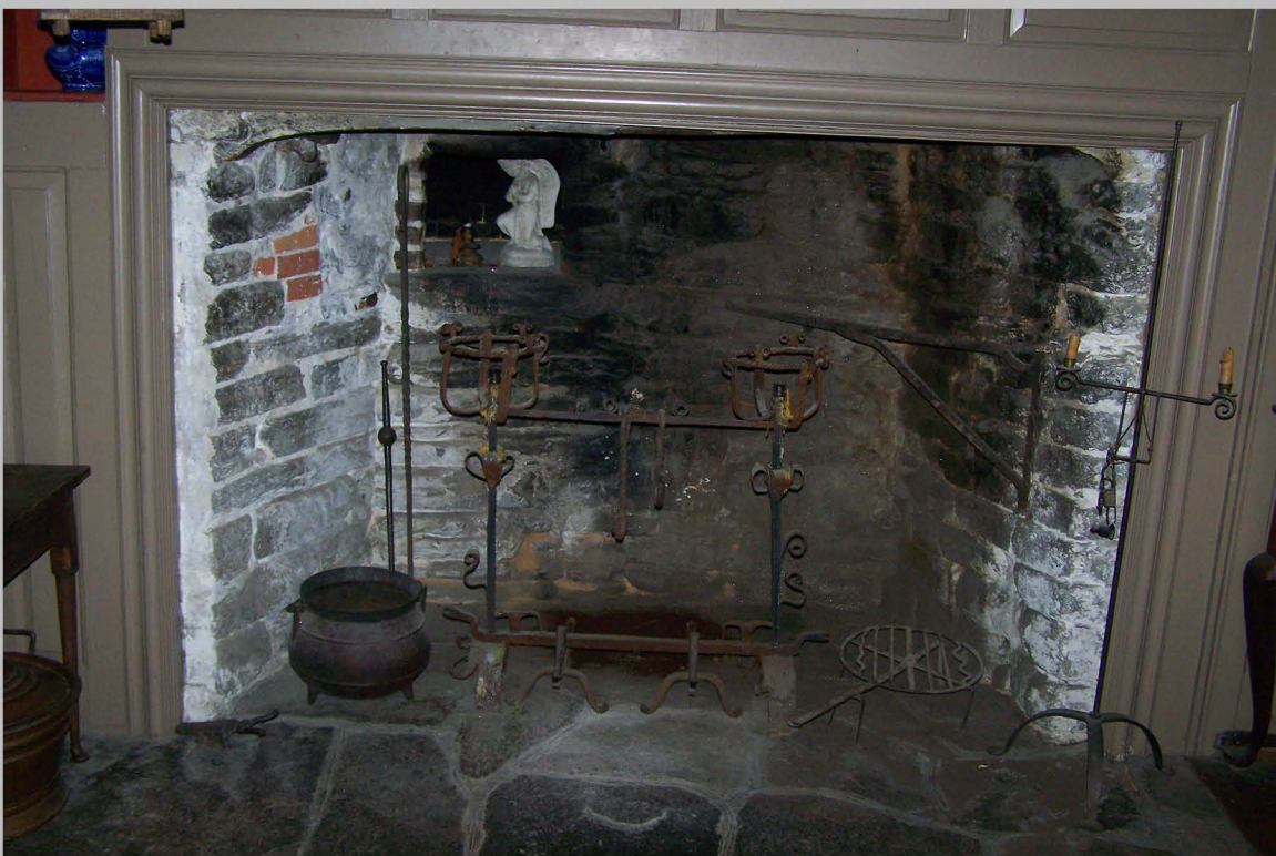
36. Main block, keeping room fireplace with oven in rear wall, view to east.
