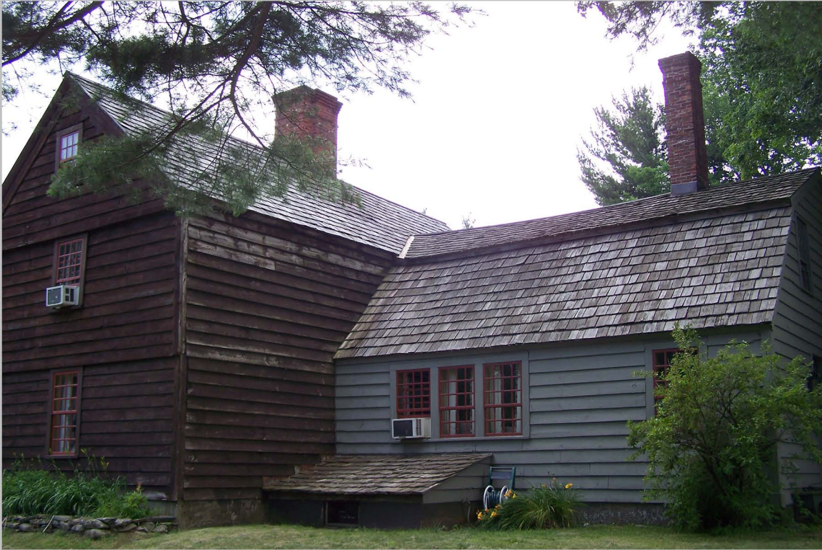
3. Main block and ell, north elevation, view to southwest.
