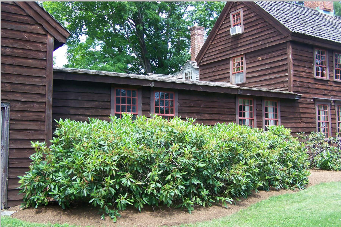
6. Wing, south elevation, view to north.
