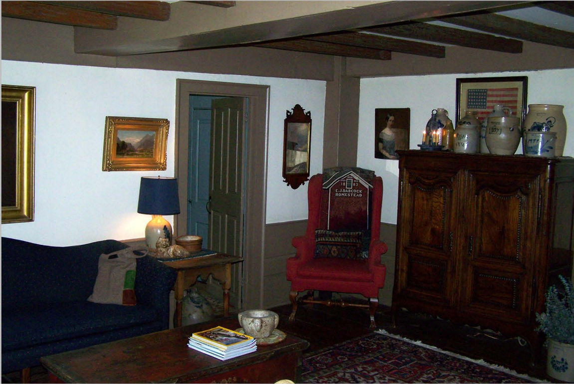
35. Main block, keeping room, cased and exposed framing and wainscoting, view to northwest.
