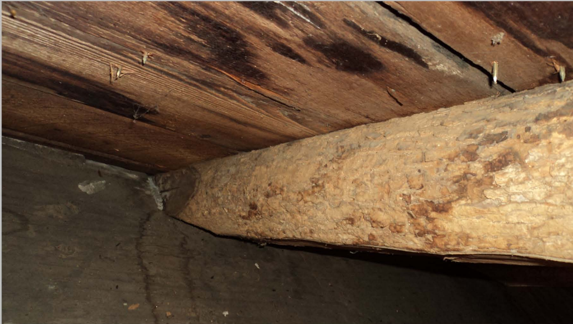
19. Attic rafter, main block, joint into plate.t
