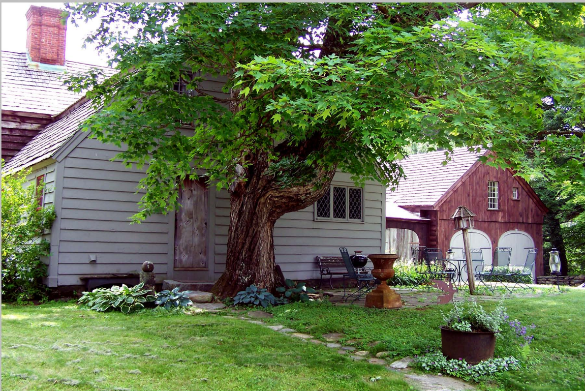
4. North elevation of ell, wing, and carriage barn, view to south.
