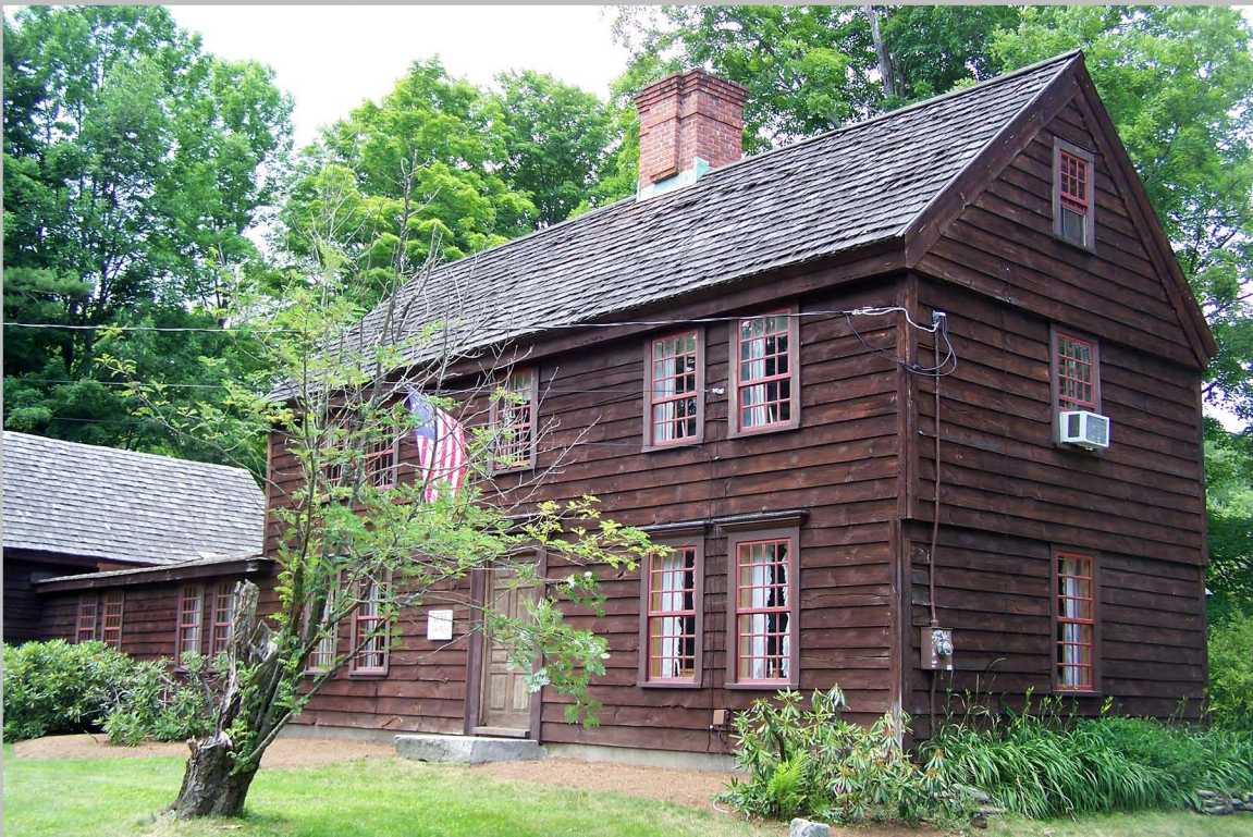
2. Main block of house view to northwest
