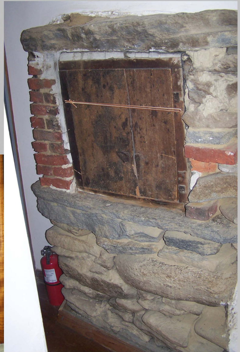
42. Main block, second floor, north side of chimney, detail of smoke oven door, view to south. (Photo: Elizabeth Rairigh, July 2014)
