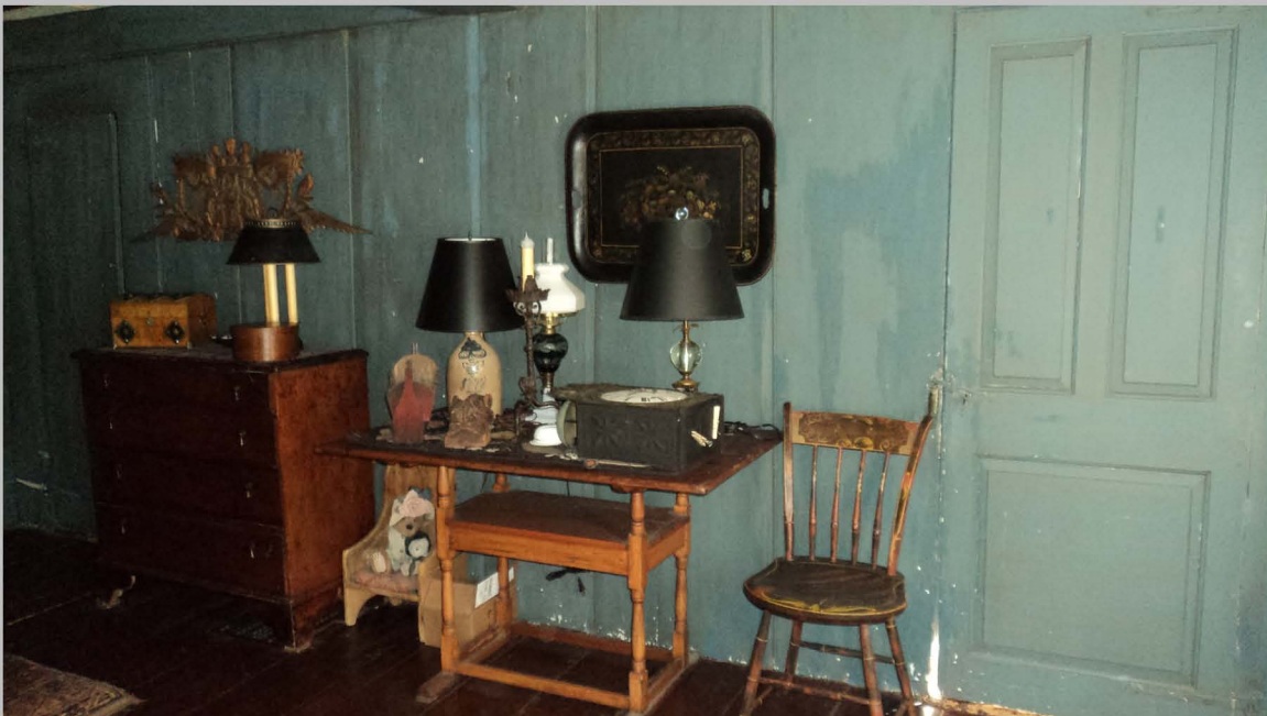
40. Main block, keeping room chamber, east wall sheathing and three-panel door, view to northeast.
