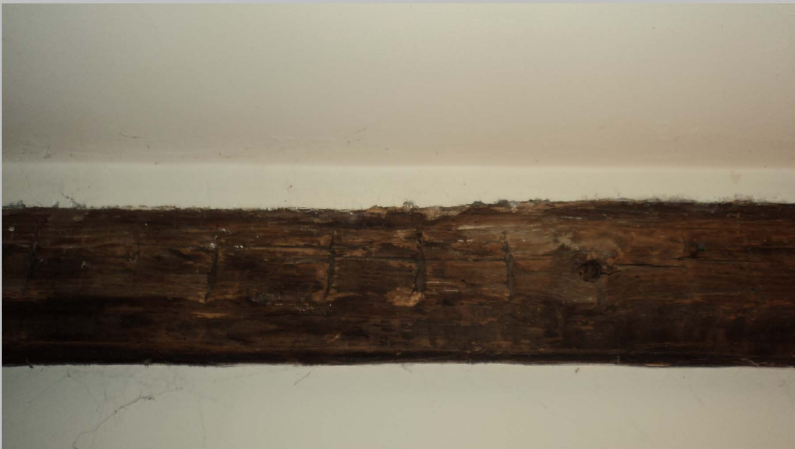
24. EII, second floor, scribe rule markings on plate, view to west.
