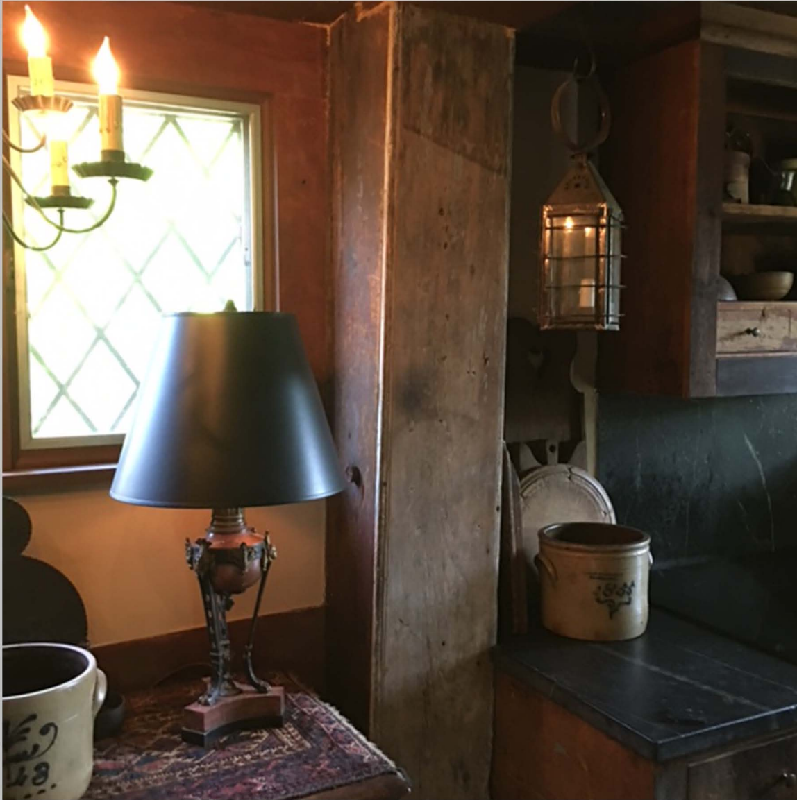
17. Cased post, ell kitchen, view to west.
