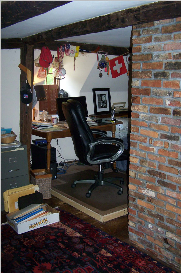
15. Ell, second floor office, view to northwest.
