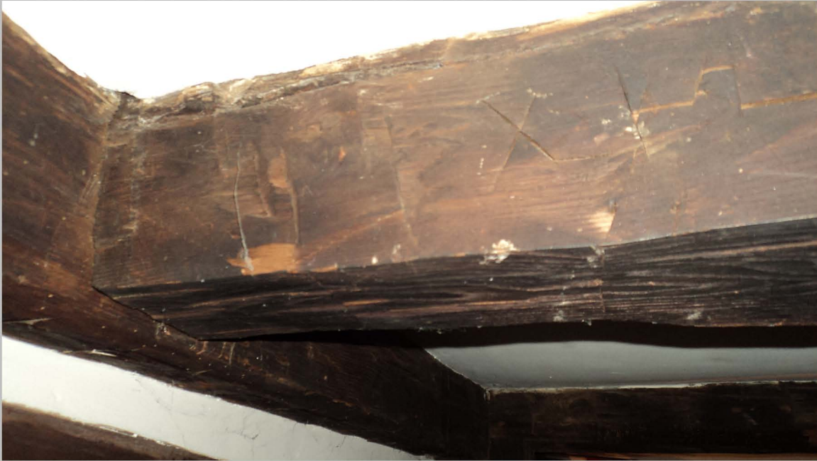
23. EII, second floor, scribe rule markings on collar tie, view to north.
