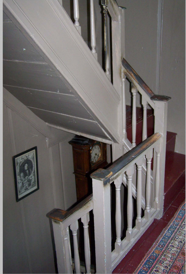
30. Main block, second floor landing, stairs and balustrade to third floor, view to northeast. (Photo: Elizabeth Rairigh, July 2014)
