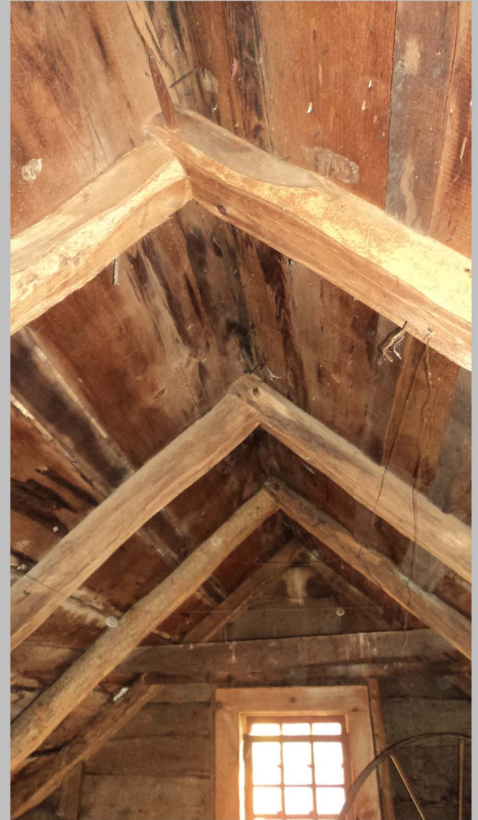
18. Attic rafters, main block, view to east.
