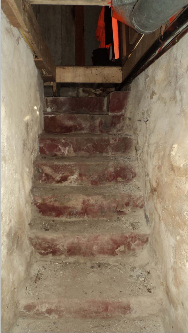
25. Ell, stairs to cellar, view to north.
