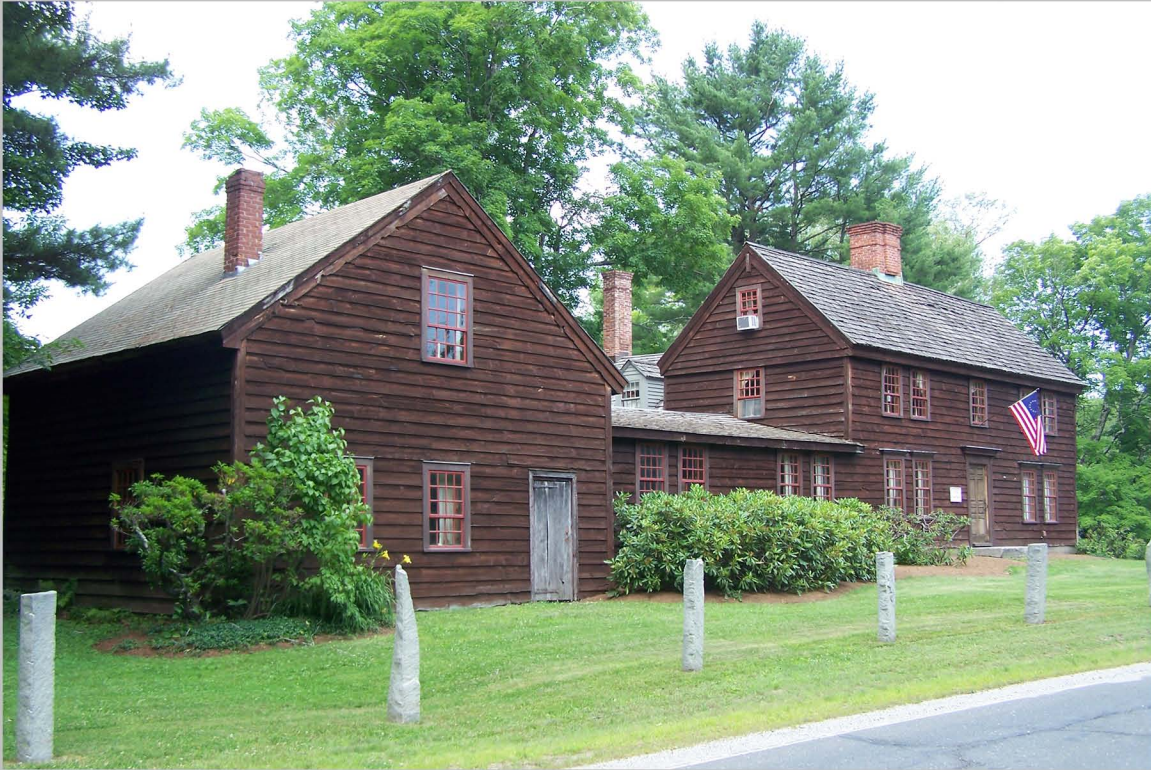
1. South façade view to northeast.
