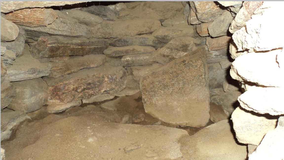
28. Main block, chimney foundation, ash pit interior, view to southwest.
