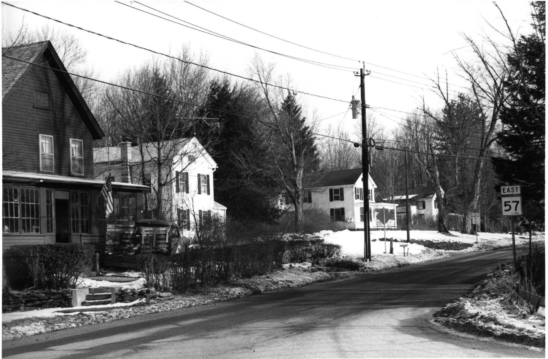
4. Looking east along north side of Main Road [at the intersection of Granby Rd and Maple St], from the west end of the Common; including the W. Moore House, GRN.69, in the foreground; the R. Barlow House, GRN.73; the second R. Barlow House, GRN.74; and the J.M. Gibbons House, GRN.79.
