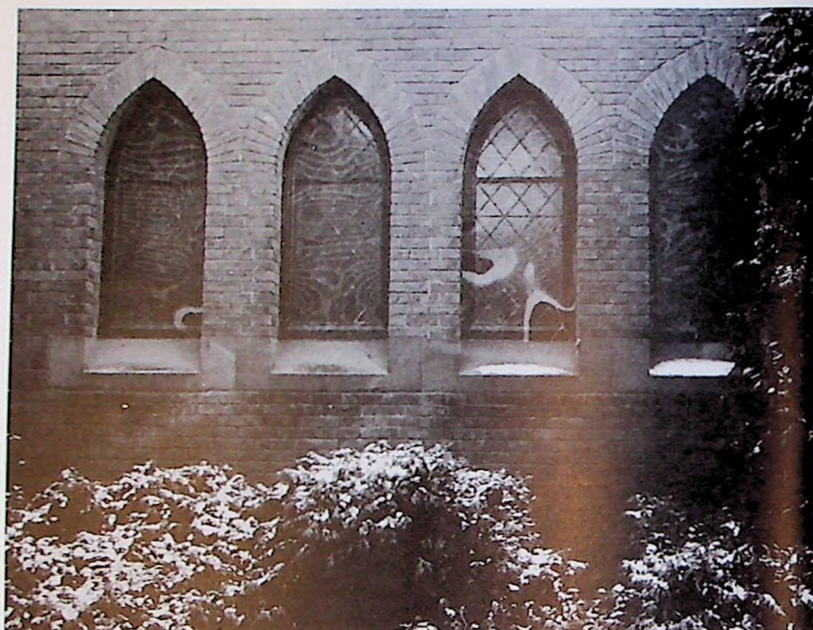
Protective plexiglass creates a ghostly effect in the windows of the Seminary chapel.
