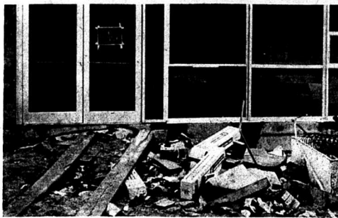
Trash and debris adorn the entrance of the newly built sports palace. Due to unfortunate delays in construction, the "No Trespassing" sign will have to remain on the door of this magnificent facility until some nebulous date in the future.
