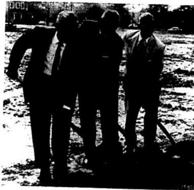
Representing their respective departments, Clifford Adams, John R. Tabb, and Admiral W. L. Messmer shovel the first ground away in preparation for construction of the new Business Administration, Physics, and Mathematics building which is scheduled to open Sept., 1962.
