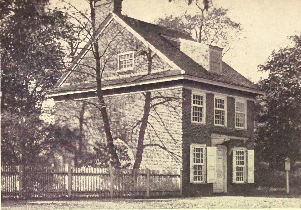
Exterior of Letitia St. House
