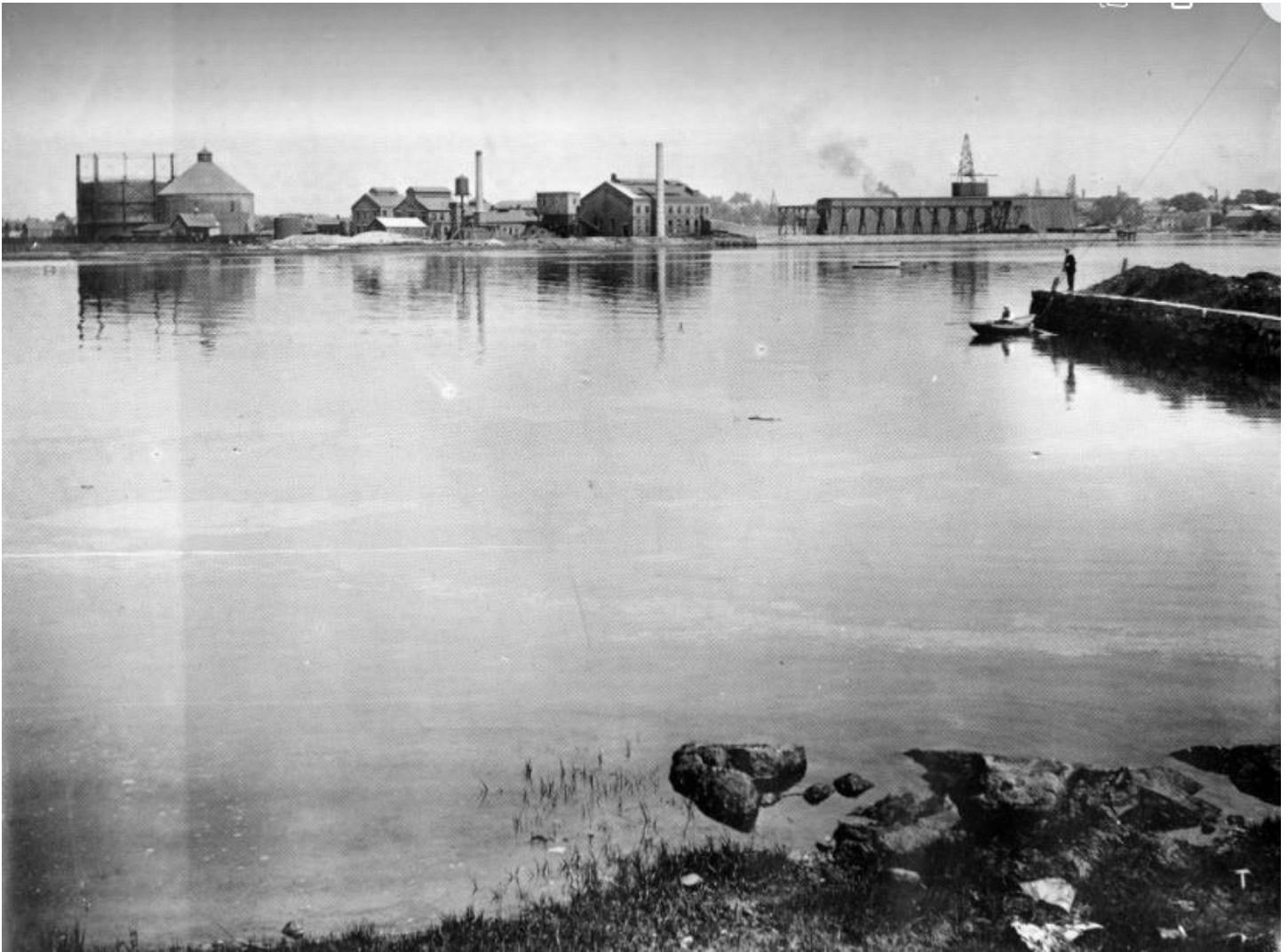
View from Collins Cove of Bridge Street Neck and Salem Gas Works
