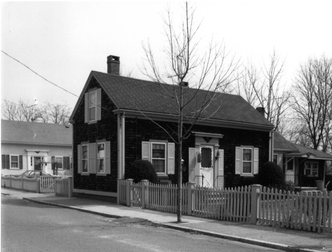
Image taken from Southwick Street Area MACRIS report: 12 Southwick, April 4, 1986.
