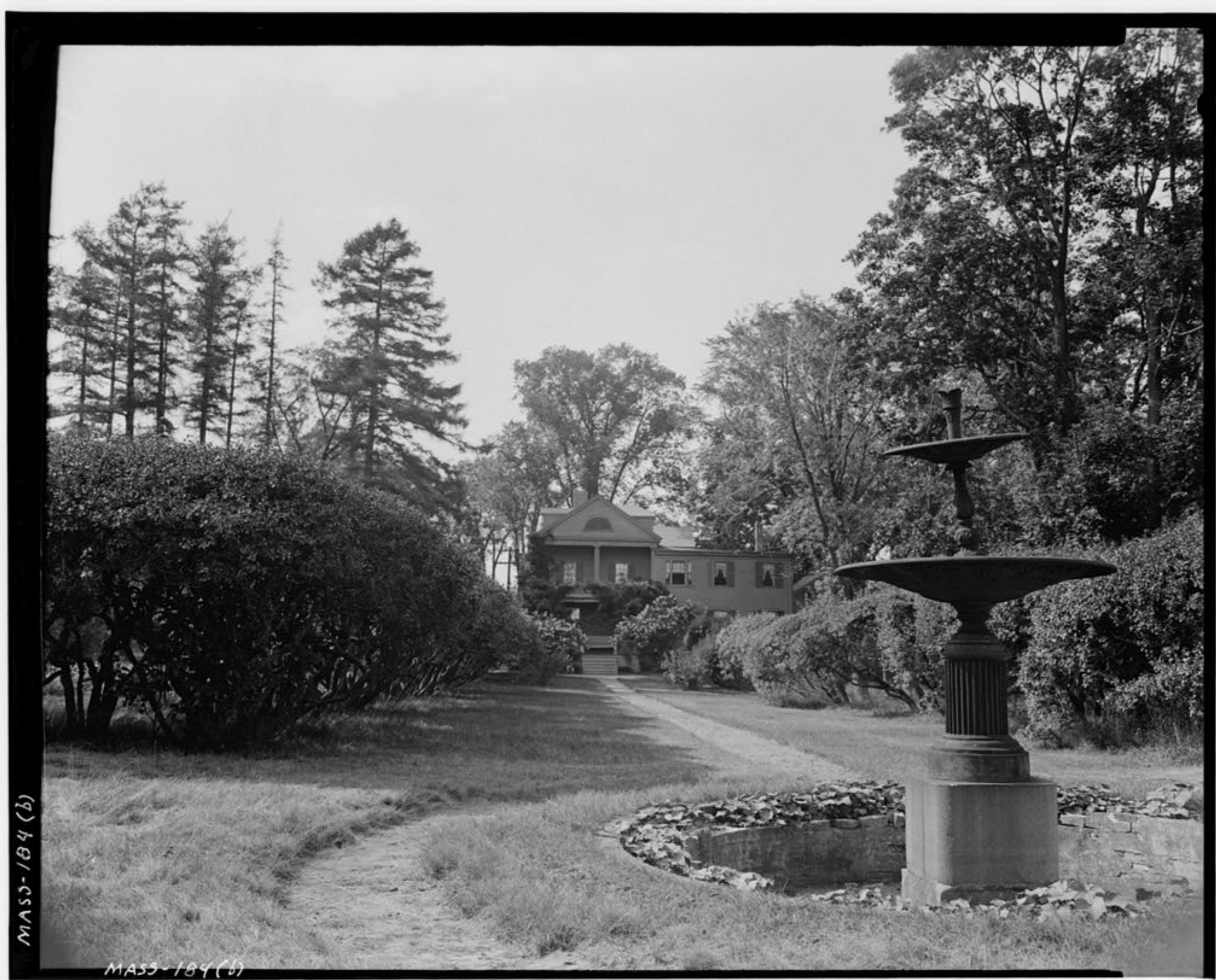
HISTORIC AMERICAN BUILDINGS SURVEY, PICKERING DODGE PLACE, PHOTO 2
