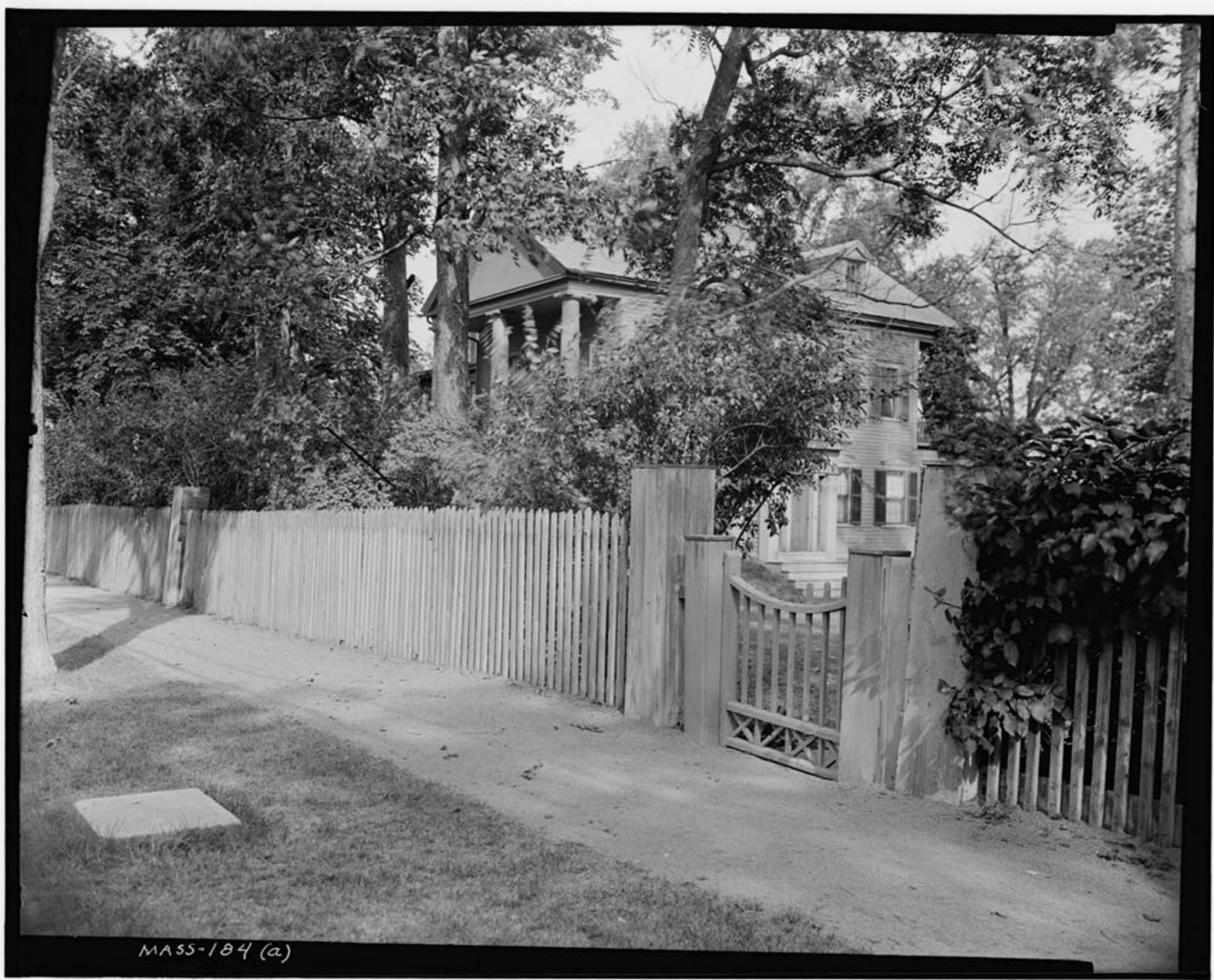
HISTORIC AMERICAN BUILDINGS SURVEY, PICKERING DODGE PLACE, PHOTO 1
