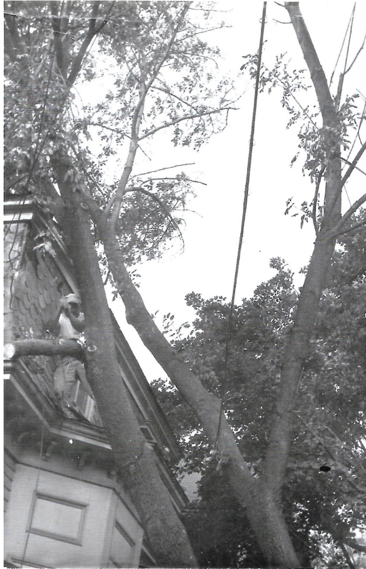
David McKay is cutting a tree away from the house after it was downed by a hurricane. Even though the McKays bought the house in 1939, it is possible this damage was a result of the 1938 Hurricane, one of the worst storms to ever hit the area.
