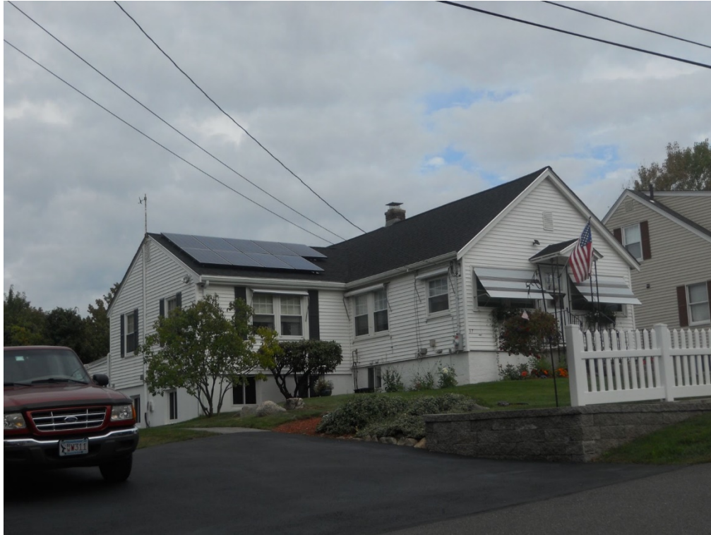
37 Clark Street, City of Salem Assessor's Office
