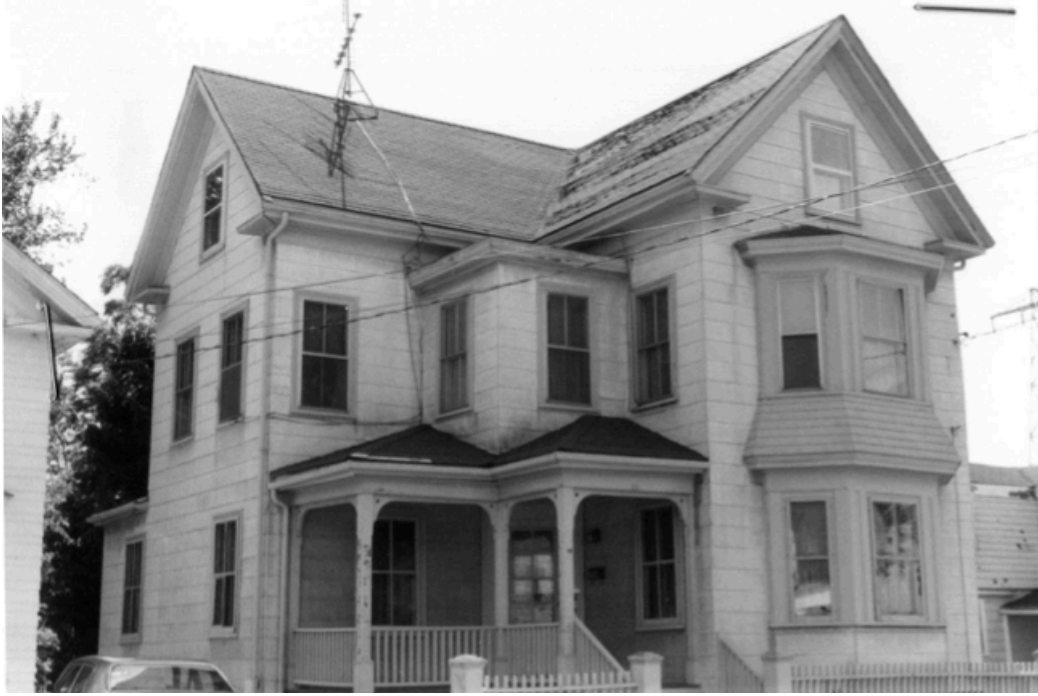
15 Thorndike St. "James J. Welch House." Constructed in 1892. Source: MACRIS SAL.3182.
