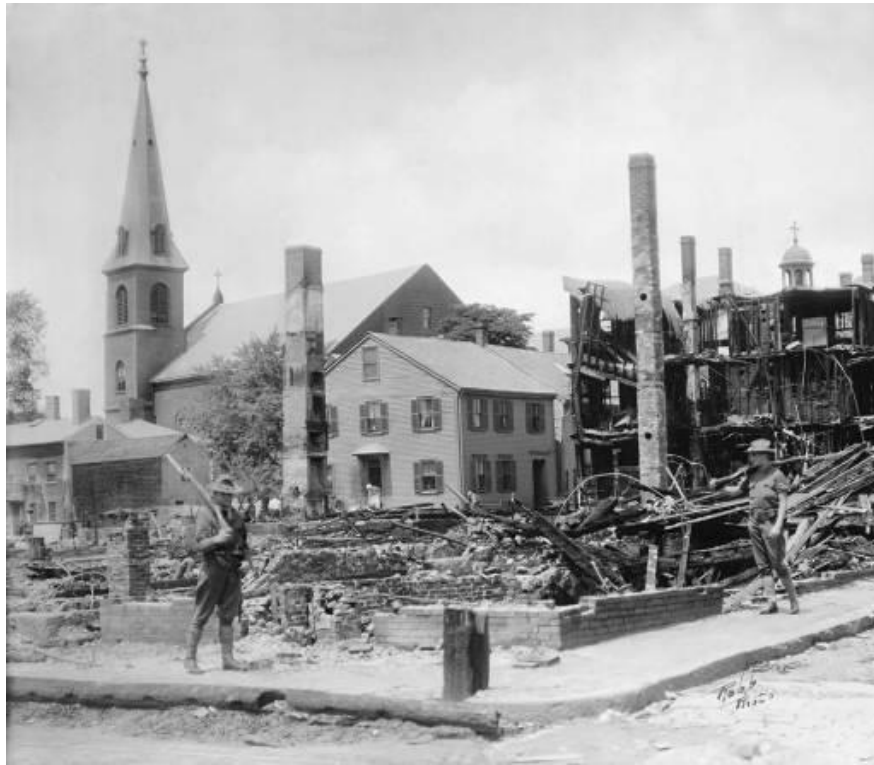
Figure 33 The edge of the fire zone at the foot of Herbert Street, with the steeple of the Polish church, by then in use as the parish school, visible just beyond the burned building and Immaculate Conception Church on the left. (Arthur Barnett Jones, The Salem Fire )
