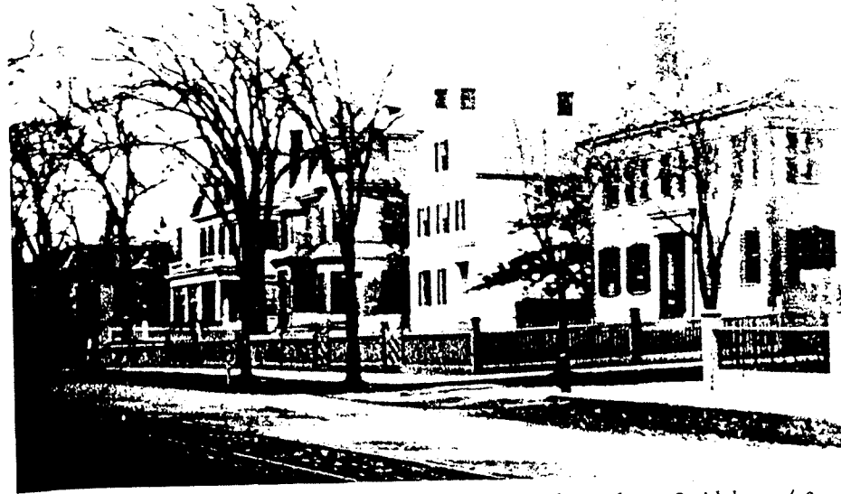
Fig. 1. John Clifton house (1848, left), 248 Lafayette Street, Salem; Alonzo Smith house (1877, left center), 244; William Pousland house (1845, right center), 244; George W. Pousland house (1843; right), 238. Essex Institute photograph, 1878.
