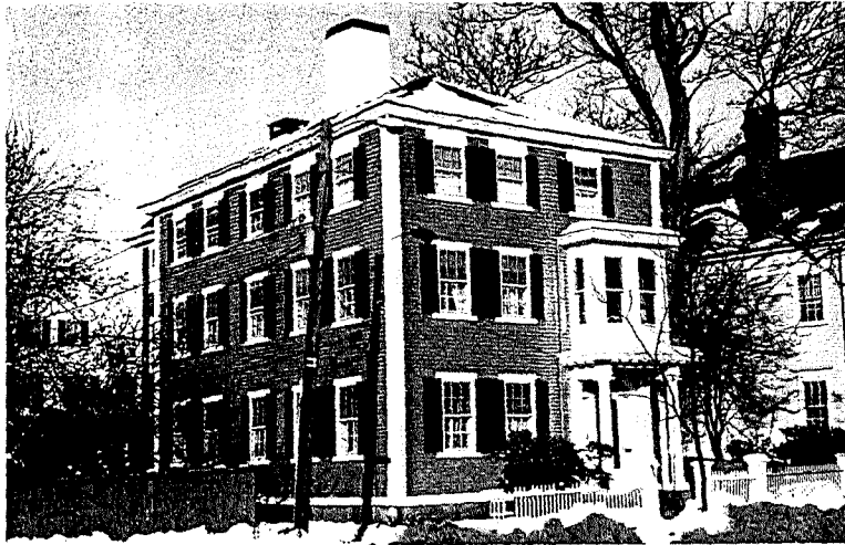
E-10 BOTT-FABENS HOUSE 18 Chestnut Street at Botts Court NR; MHD
