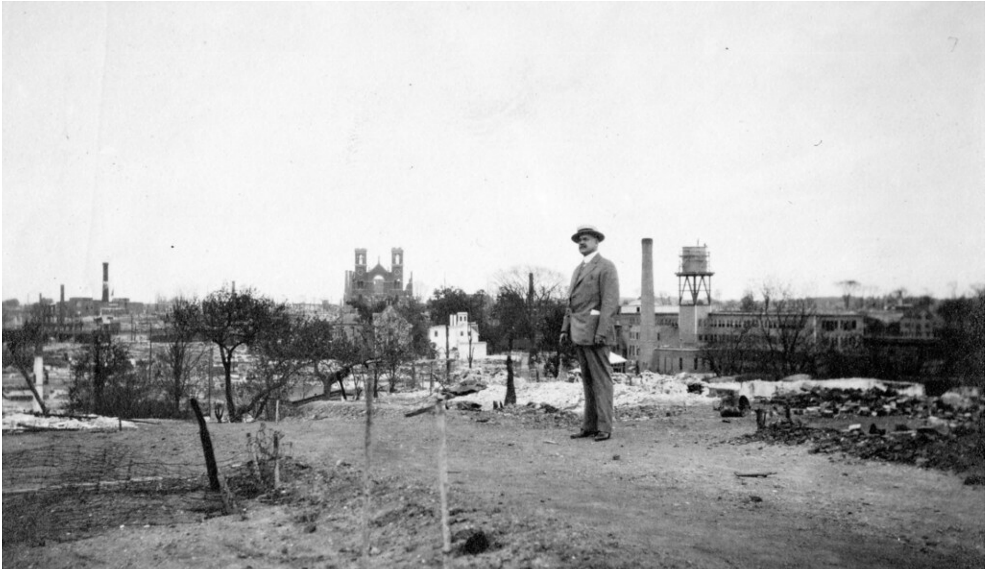
Man poses among the ruins of the Great Salem Fire of 1914. Likely taken near Phelps Street. St. Joseph's Church at 135 Lafayette Street in the distance. On back "General view of burned district" SCPH 13-018 Salem State University Archives and Special Collections
