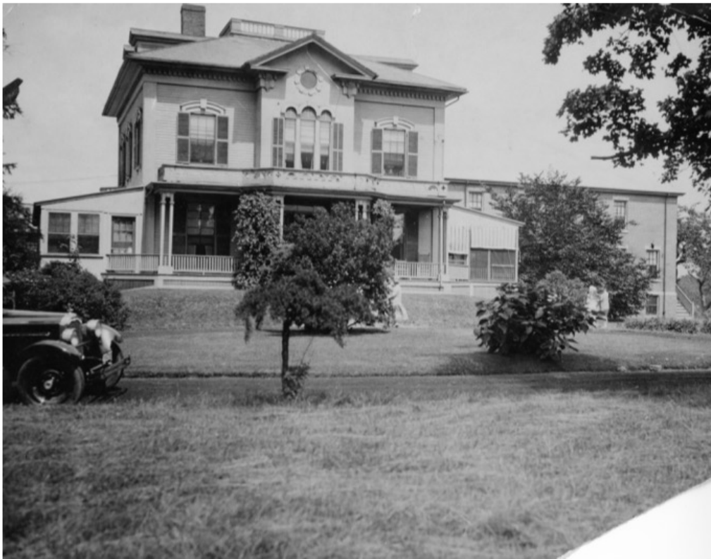
Charles A. Ropes house, later North Shore Babies Hospital, c. 1856, no longer extant. 1927 image, Salem State University Archives. The long ell at right was a c. 1926 addition; the flanking shed roof wings on either side of the main house were added c. 1909, as "fresh-air wards" for the young patients.
