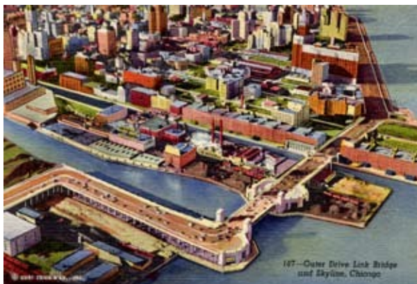
The 1937 Lake Shore Drive Bridge was built in the moderne style, not the classical look favored by Bennett.
