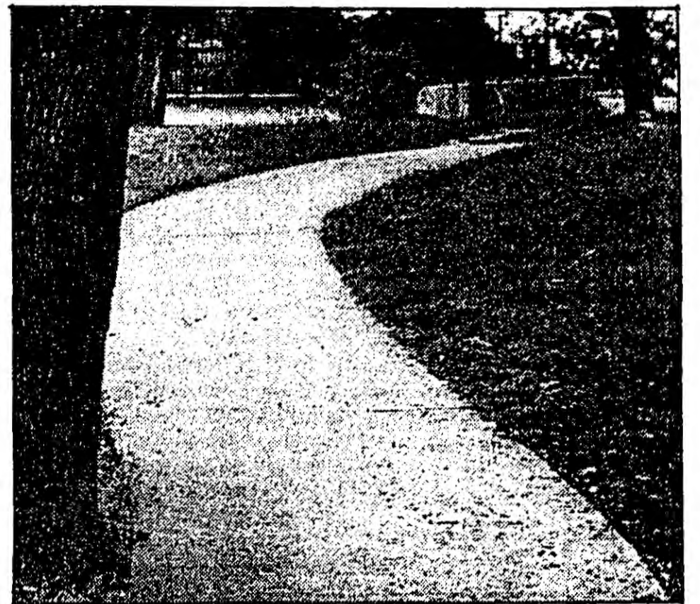
OLD HANDICAPPED RAMP, which is found too steep and dangerous, is being replaced by the new elevator. (Photo by Marc Mormino)
