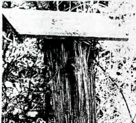
SIGN POST WITH NO SIGN--Weather and vandals have contributed to the destruction of markers along the nature trail. Repairs for them will begin soon.
