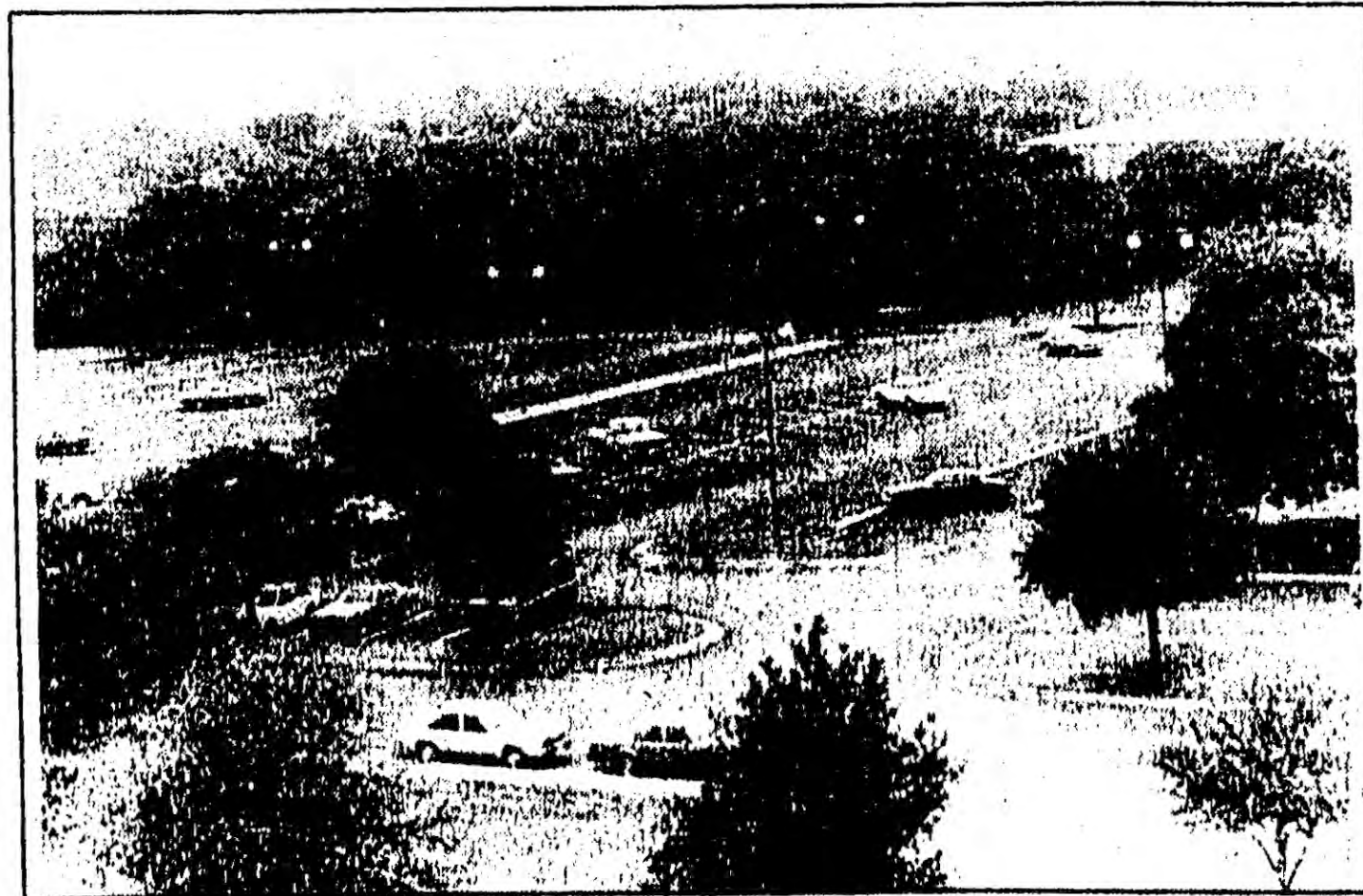
MCC PARKING LOTS, which have undergone extensive reconstruction during the past few months, are still in need of certain types of work. Repaving and parking lines still are needed in some places. (Photo by Marc Mormino)
