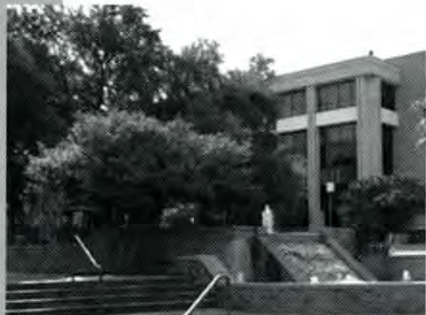
Administration/ Classroom building
