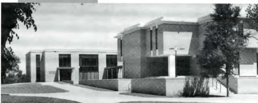
Liberal Arts and Faculty Offices buildings
