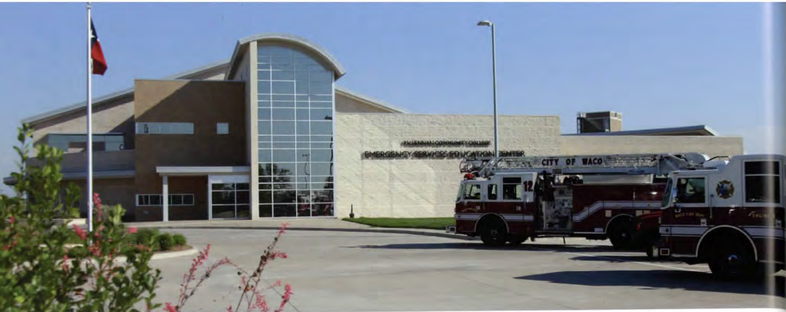
The multidiscipline Emergency Services Education Center generated substantial media and community interest when it opened in 2009.
