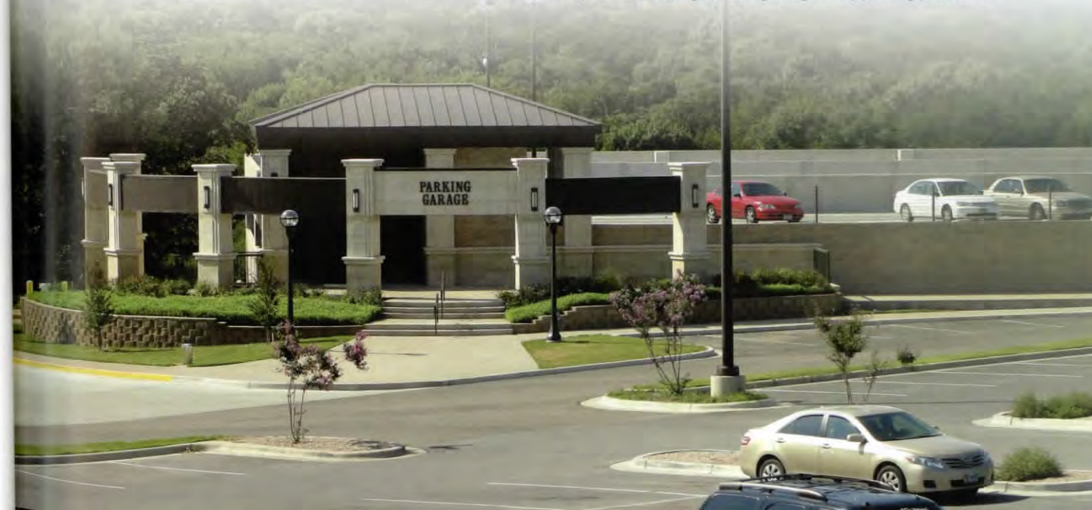
The 400-space Highlander Drive Parking Garage opened in August 2009 as the first step toward solving the college’s legendary parking problems.
