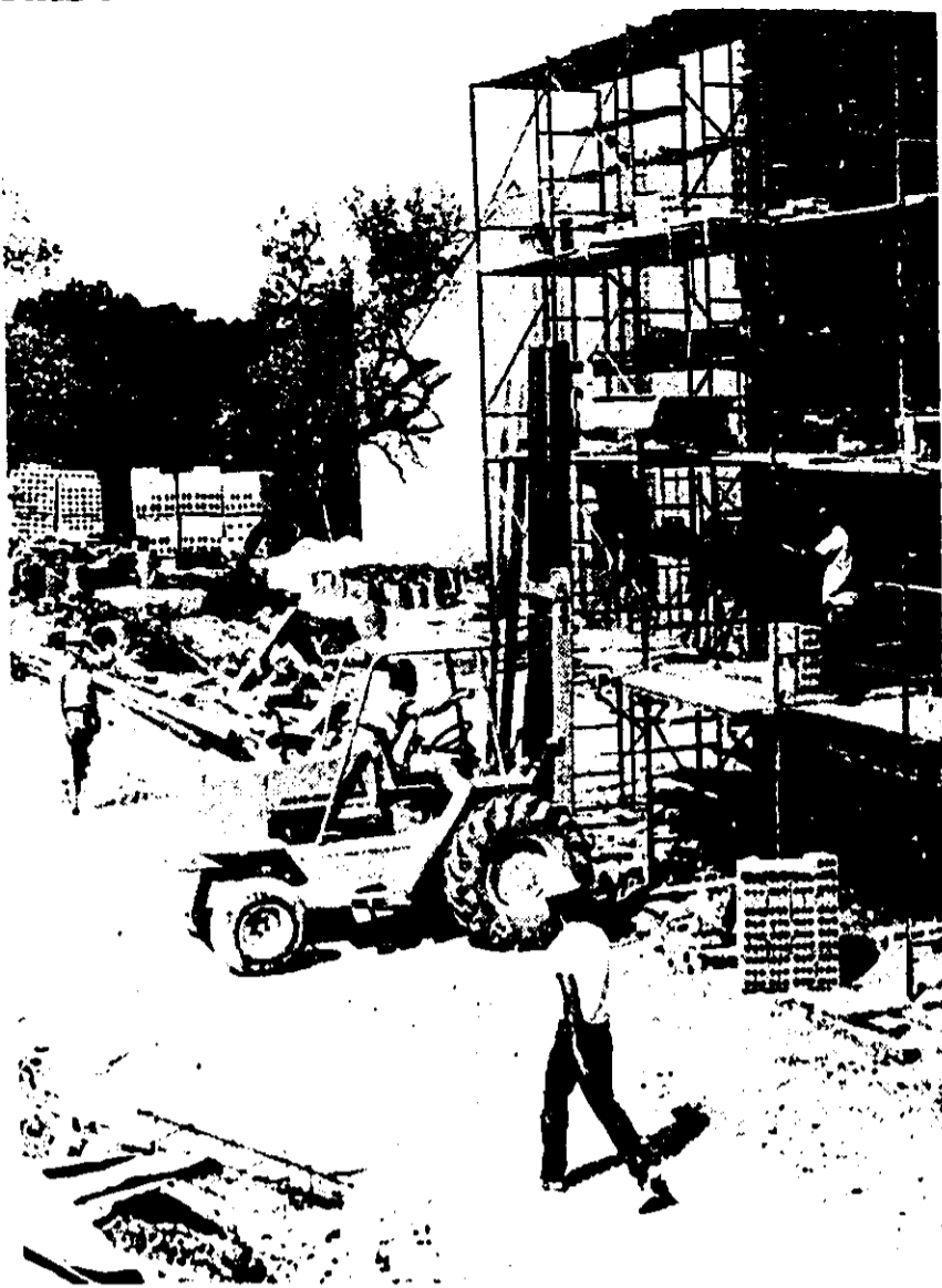
WORK CONTINUES on the Health and Physical Education Center, which is due for completion this fall. The modern facilities will include gym, lounge area and classrooms. Waco Construction, Inc. are general contractors for the center.
