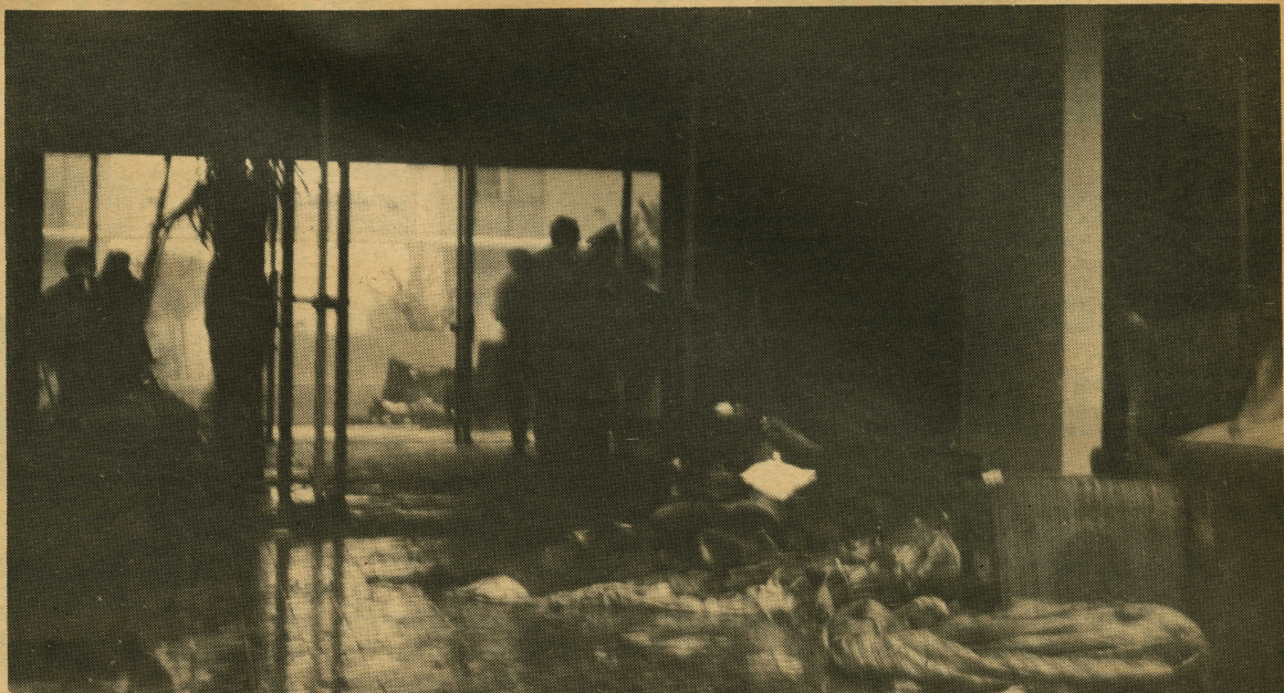
MEAD RUBBLE-- Charred lobby of Pitzer's Mead Hall after arsonist did his work. Dam-
