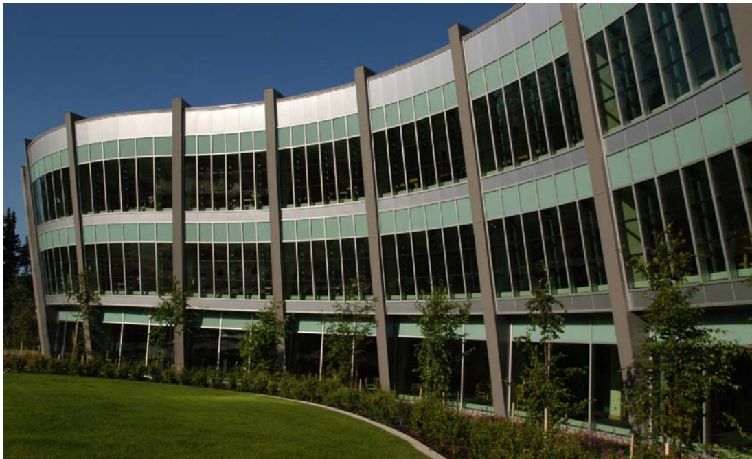
Fig. 2. Serpentine exterior wall of Consortium Library.
