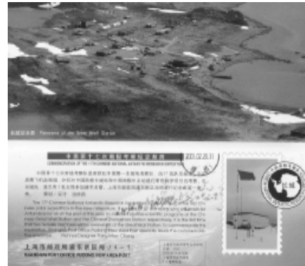
Above: Postal cover showing Great Wall Station as seen from the air at the end of the season in 2001.
