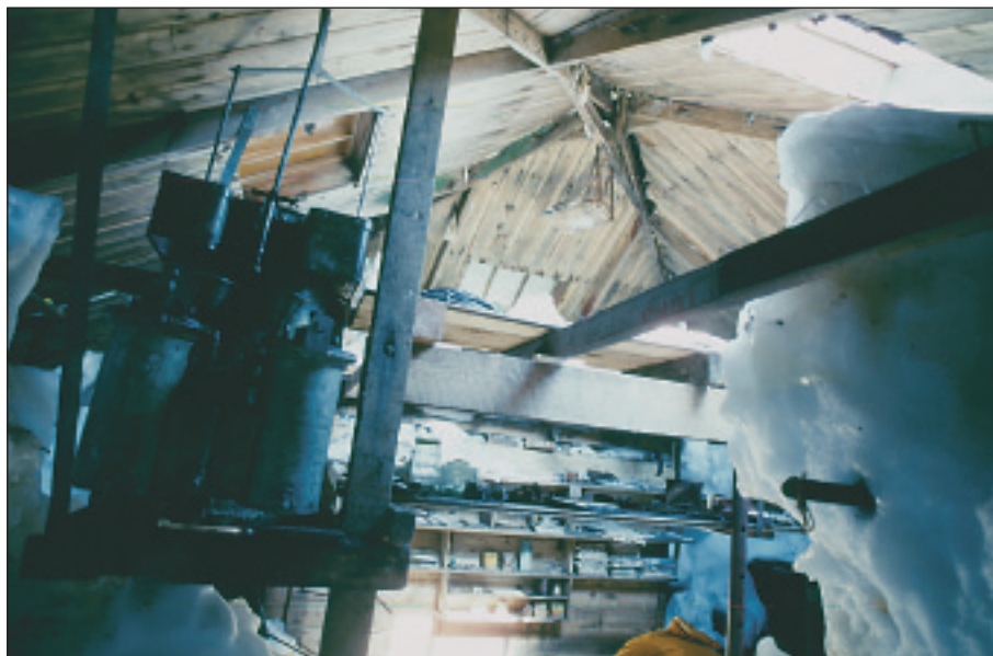
Interior of the main hut showing ice accumulation surrounding bunks and storage platform. In the left foreground is the acetylene plant used for lighting. ROB EASTHER
