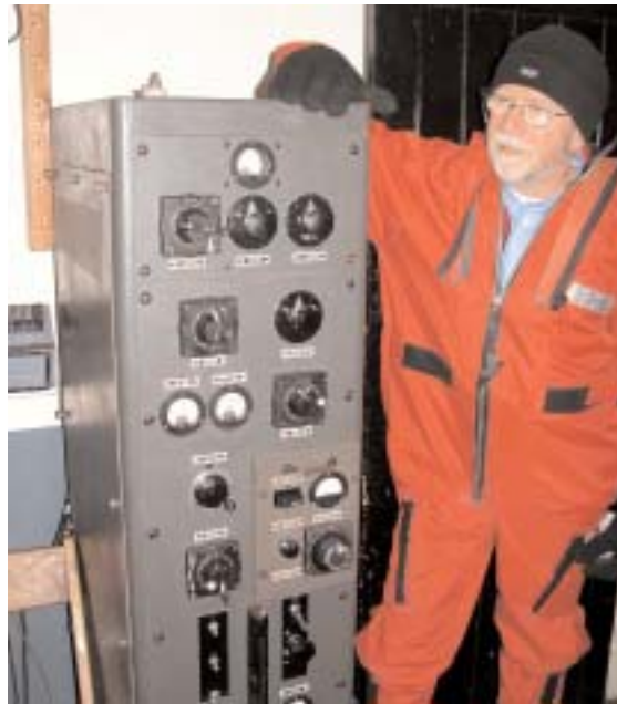
Radio equipment at Horseshoe with Tom Maggs (Australia).
