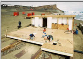
Construction of the Czech Station
