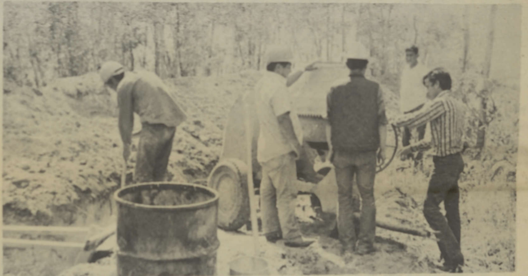
Installing manhole for sewer.
