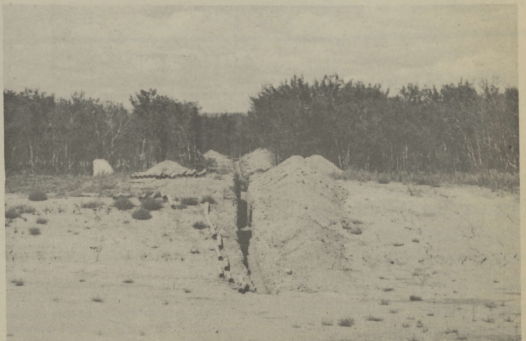
Sewer ditches nearly completed.
